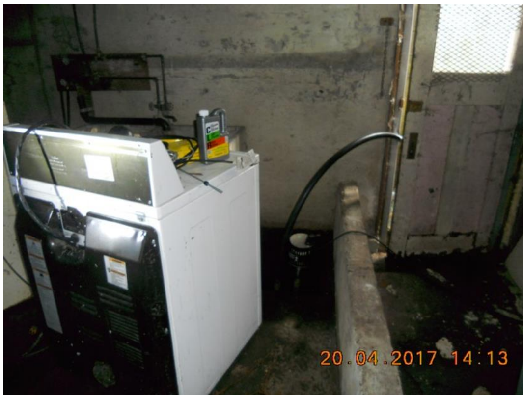
Basement - washer unit not operational, sump pump operating and pumping water out basement door into neighbouring property located at 507 - 11th S (owned by Bell, JW)
