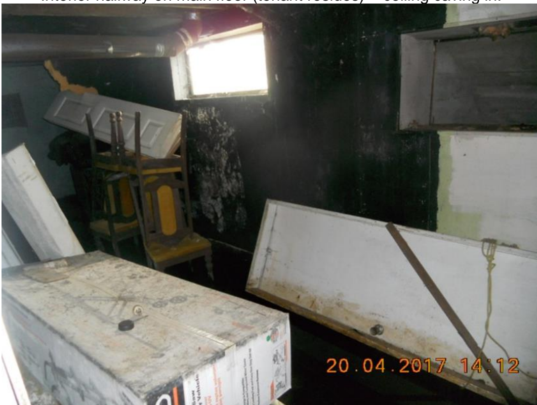
Basement - broader view of area with water accumulated, furniture stored, black mold
