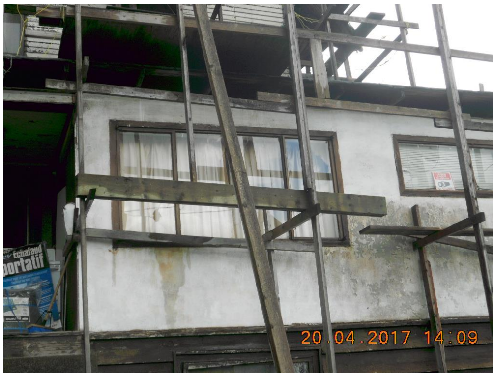
April 20, 2017: Broken front window, water damage on stucco
