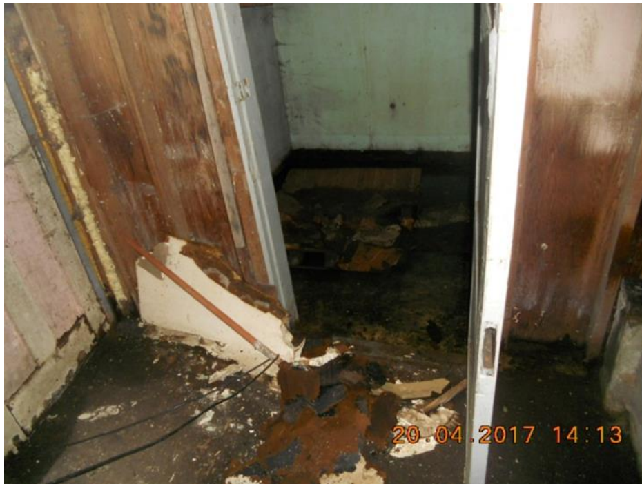
Basement - water damage, mould on floor, walls, frames
