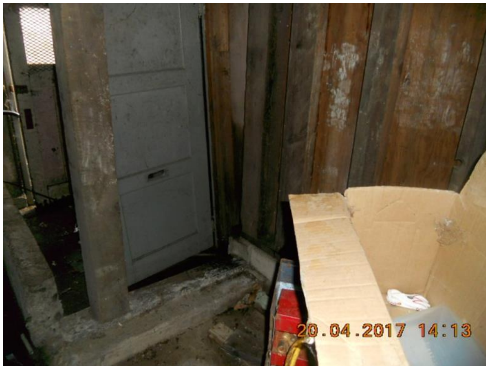
Basement – mold on walls & beams
