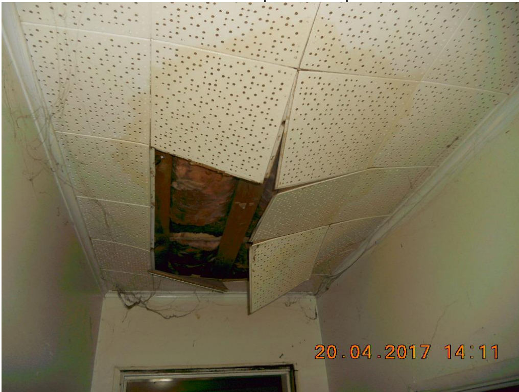
Interior hallway on main floor (tenant resides) – ceiling caving in.
