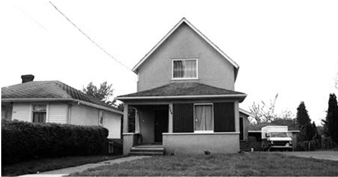
The subject house in 1982. Source: NWMA IHP14365
