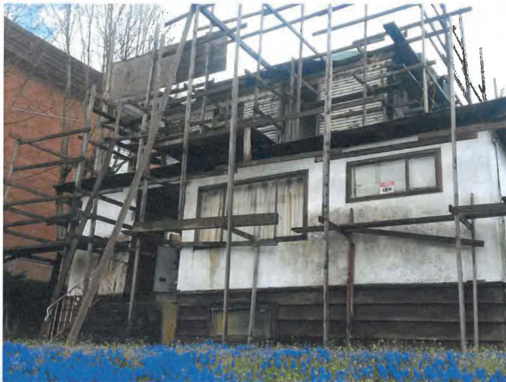
Figure 1 West Elevation – Windows Removed From Top Floor
