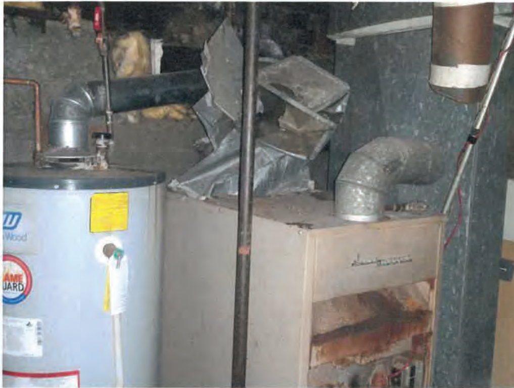
Figure 5 Basement -- Furnace Has Been Disabled
