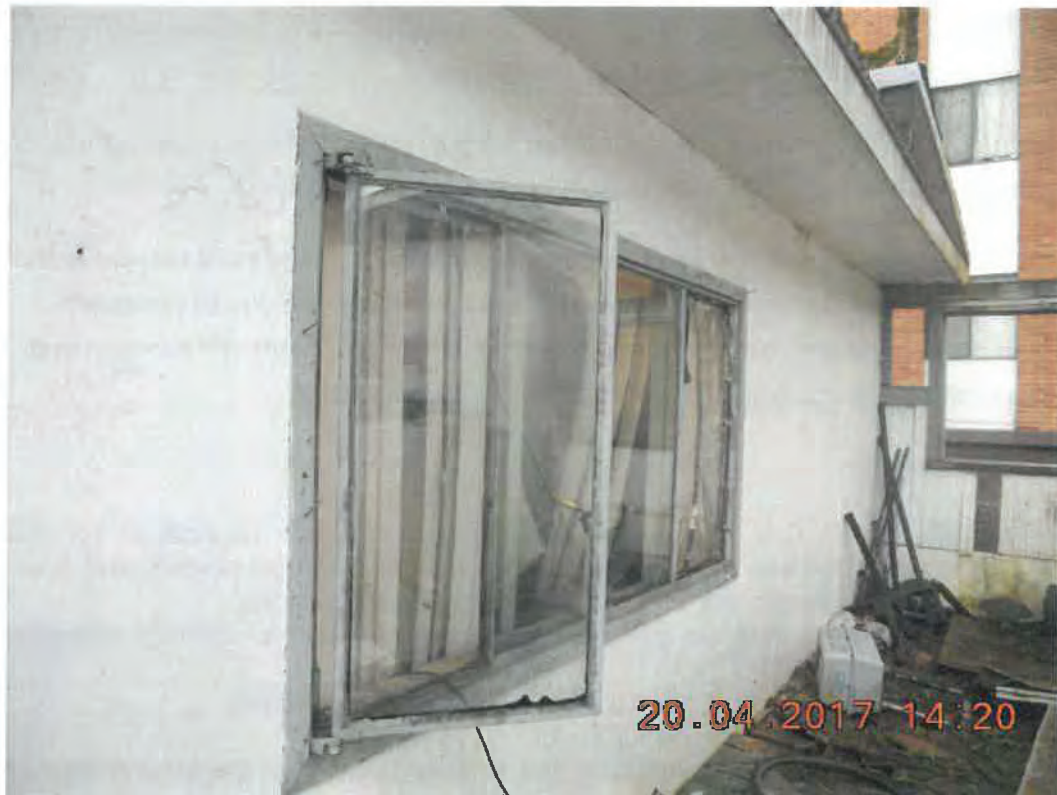
Figure 11: Rear - broken window into living area
