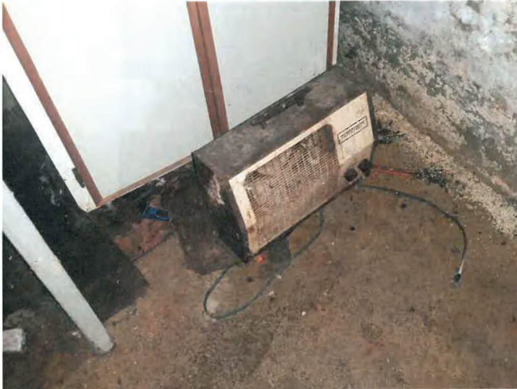
Figure 6 Basement -- Use of a Temporary Heater for Primary Heating
