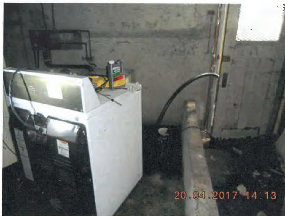
Figure 8: Basement - sump pump operating and directing water into neighbouring yard
