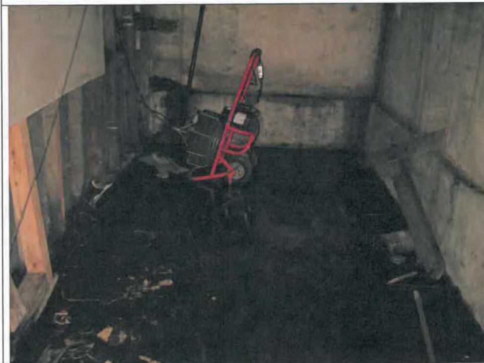
Bottom of studs are wet
