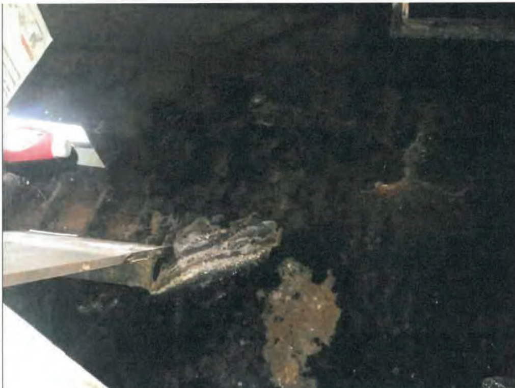
Figure 3 Basement floor towards the West Elevation -- Pool of Stagnant Water
