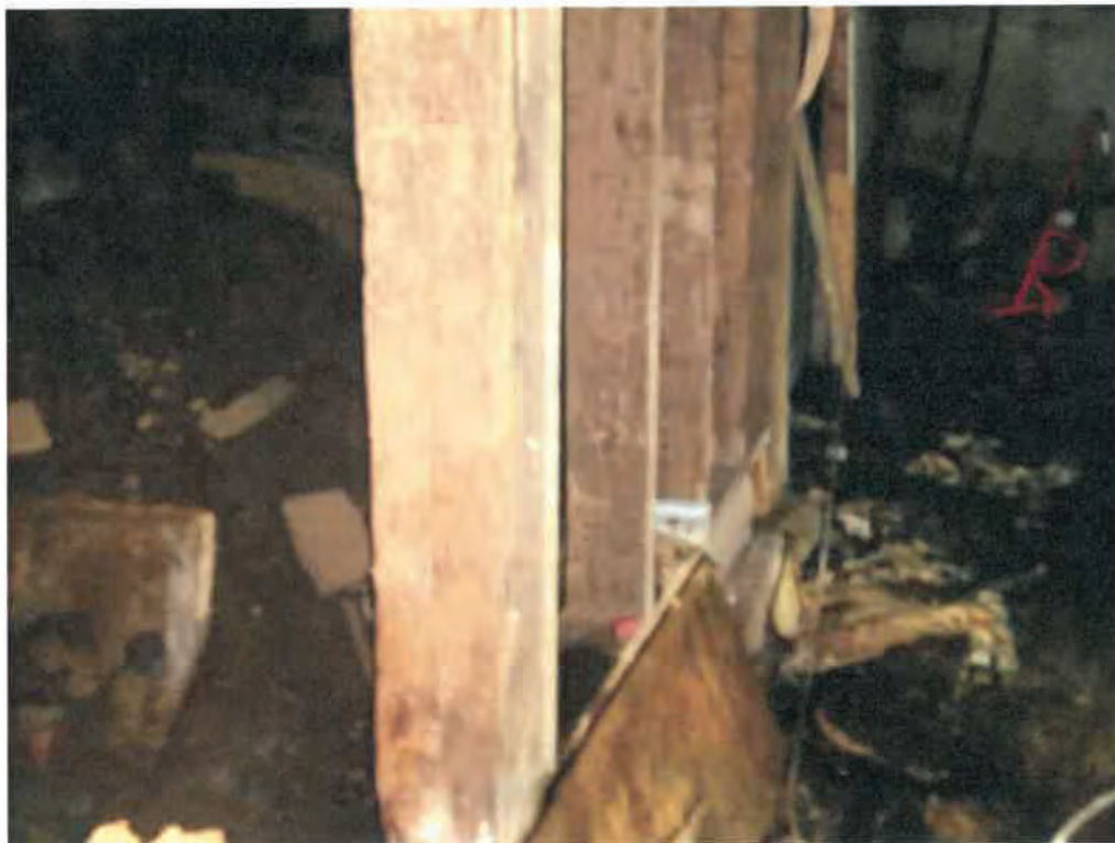
Figure 7 Basement -- Debris and Wet floor -- Black Mold Present
