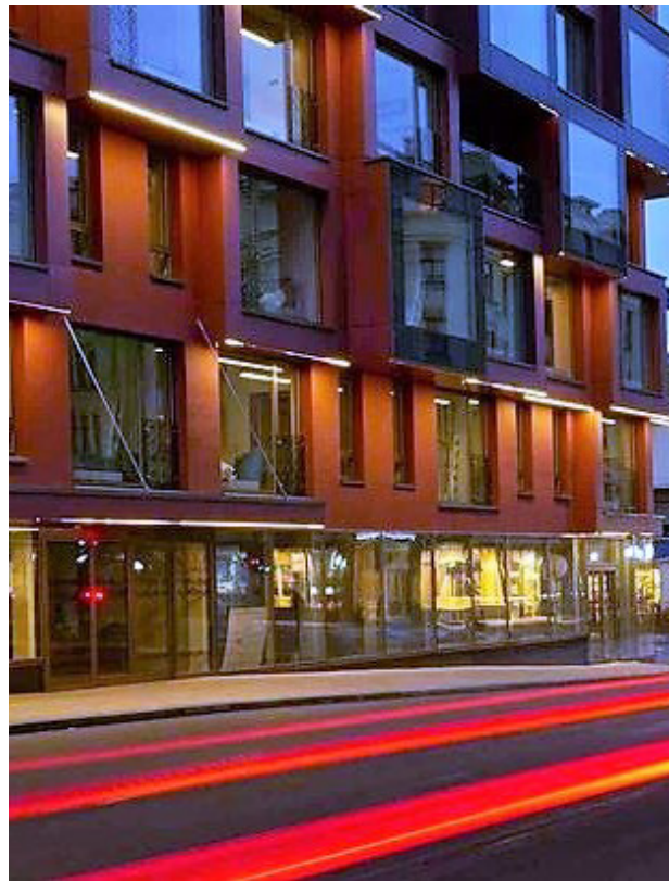
Lighting as a feature element integrated into the façade, Source: NRJA Architecture
