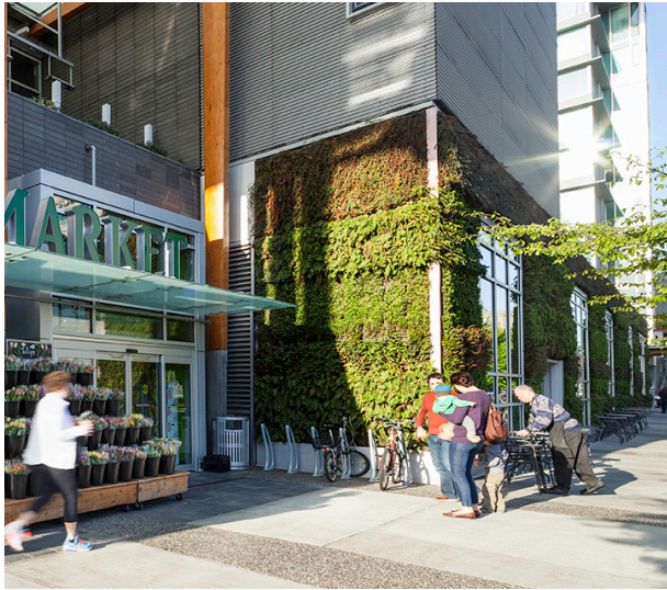
Details like a green wall can enhance public realm along a street frontage, Source: Perkins+Will
