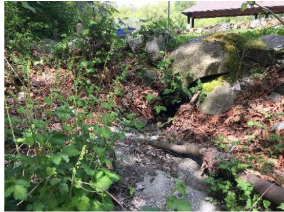
View of culvert under Hume Park Rd
