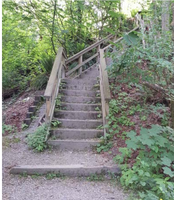
Figure 16 – Stairwell connecting lower (south) and upper (north and west) areas of the park
