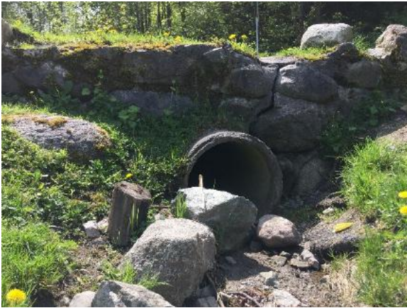
View of culvert below Hume Park Rd
