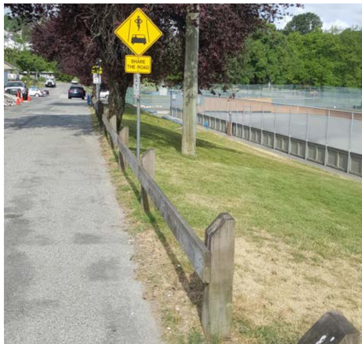
Figure 12 - No sidewalks on north side of Garrett Street
