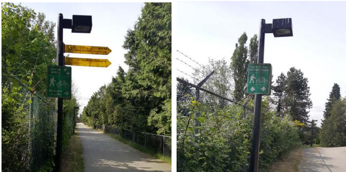
Figure 17 – Examples of faded and weathered wayfinding signage
