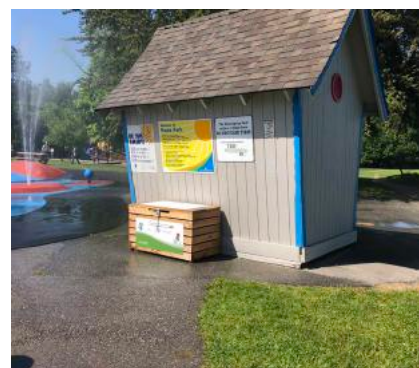
Spray Park Service Building
