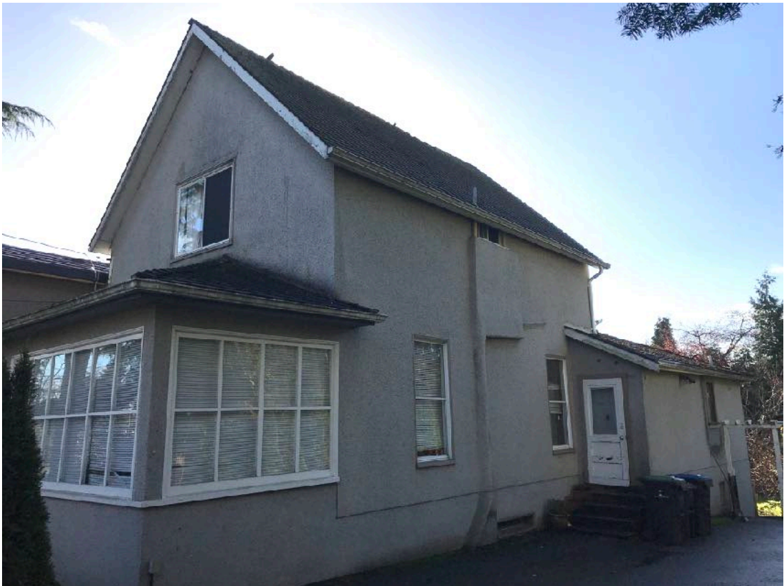
Below: side (northwest) elevation
