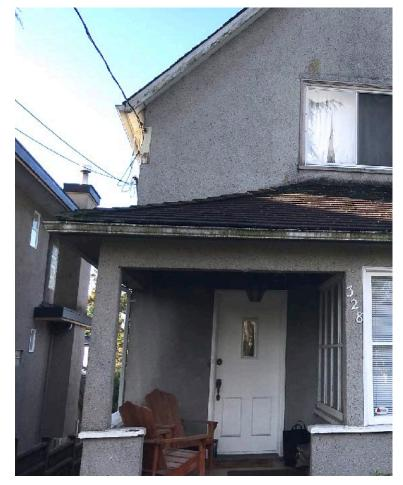
in mid-century (the earliest documentation of its presence is in 1967, in a City field inspection report) is showing signs of moisture ingress at various points around the building and is thus considered to be in **fair** condition. The spot deterioration of the stucco will have allowed
