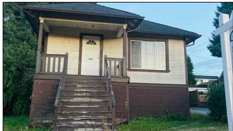
EXISTING HOUSE AT FRONT STREET
