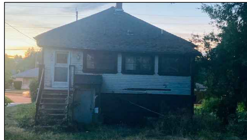
EXISTING HOUSE AT REAR LANE
