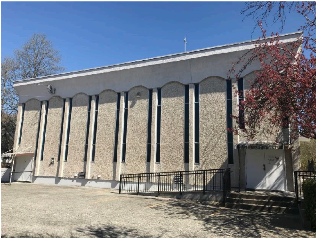
Side view (facing parking lot)
