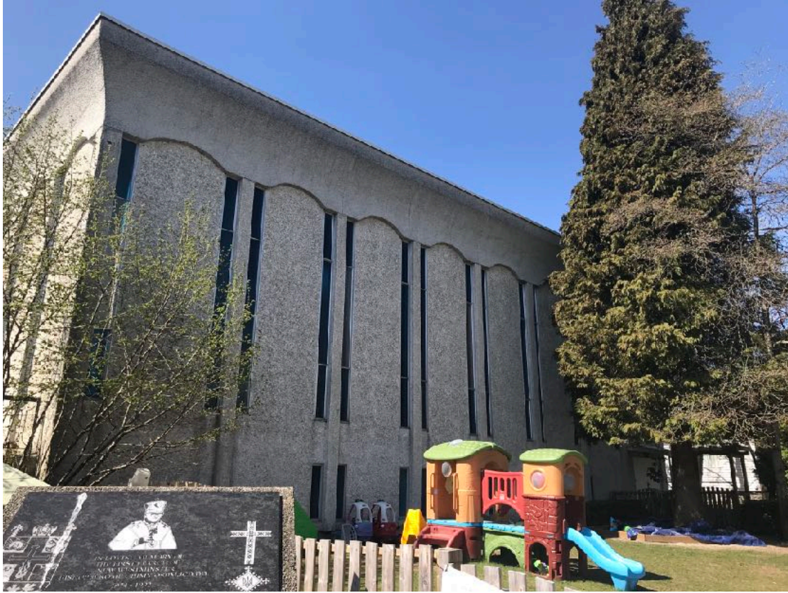
Side view (facing 5th Street)
