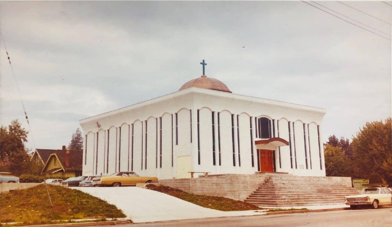
Early photograph of the recently completed Holy Eucharist church, circa 1969. Source: Holy Eucharist Cathedral Parish Archives
