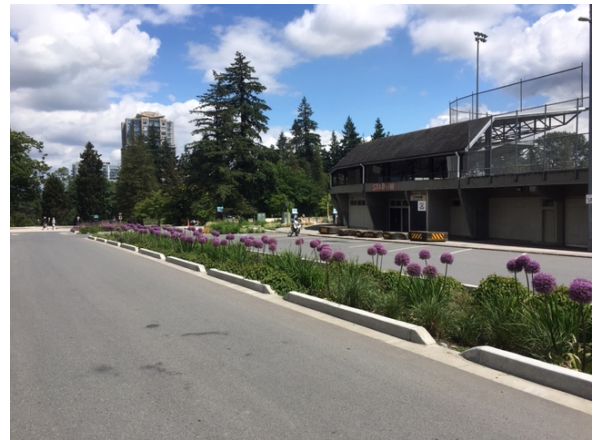
Photo 43 A rain garden installed in a new parking lot in Queens park.
