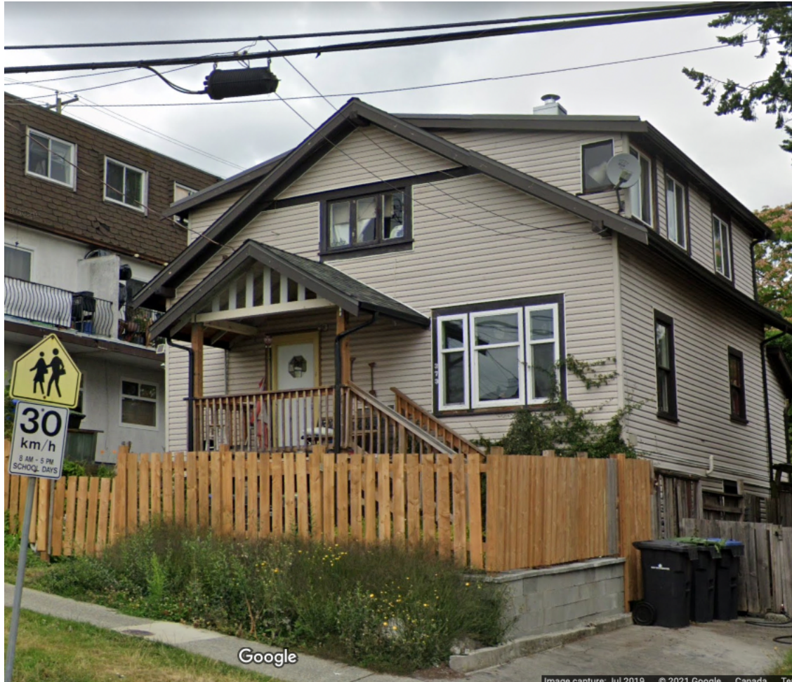
2019. Google. (Note: Front porch partially rebuilt, wood transomed window combination replaced with vinyl windows, brick chimney replaced with metal chimney.)
