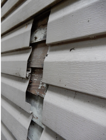
Wood lap siding on north elevation under vinyl siding.
