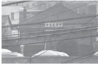
South Elevation of former Chinese Benevolent Association building (Courtesy New Westminster Archives)
