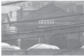
South Elevation of former Chinese Benevolent Association building (Courtesy New Westminster Archives)
