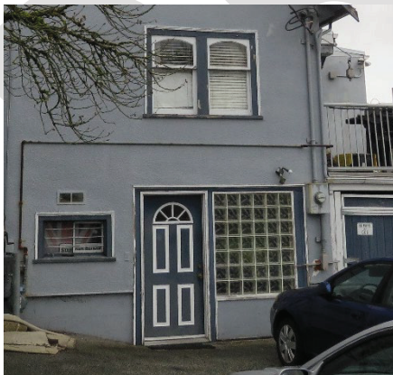
Non-historic windows, before replacement (March 2020)
