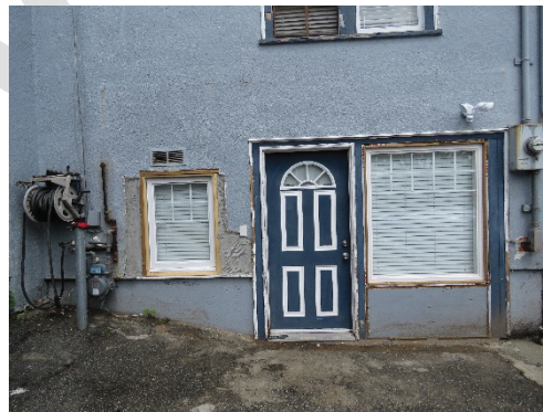
Replacement windows. (July 2020)
