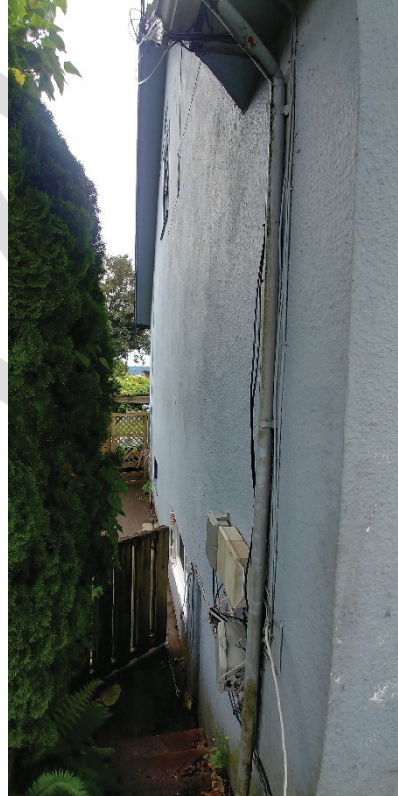
Side (northeast) Elevation
