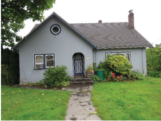
Front (northwest) Elevation
