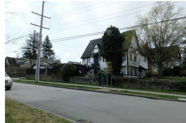
HERITAGE HOUSE FROM NORTH WEST
