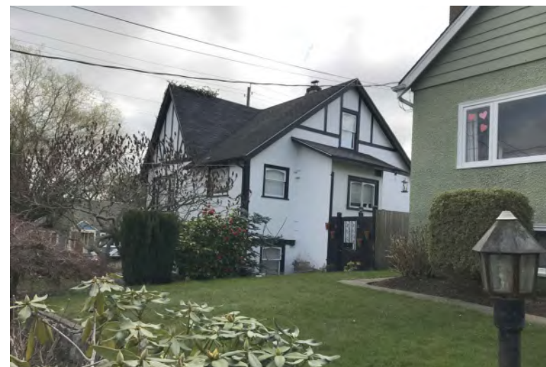
HERITAGE HOUSE FROM NORTH WEST
