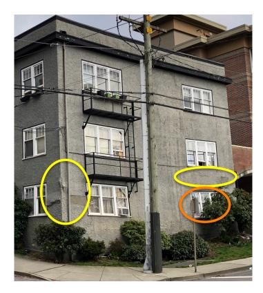
Figure 18: Cracking, buckling and spalling of stucco (yellow highlight), buckling of window frame (orange highlight)
