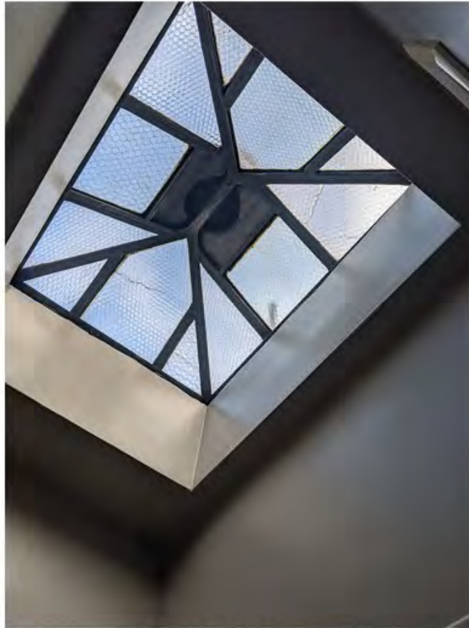
unit 351 - skylight with cracking.jpg
