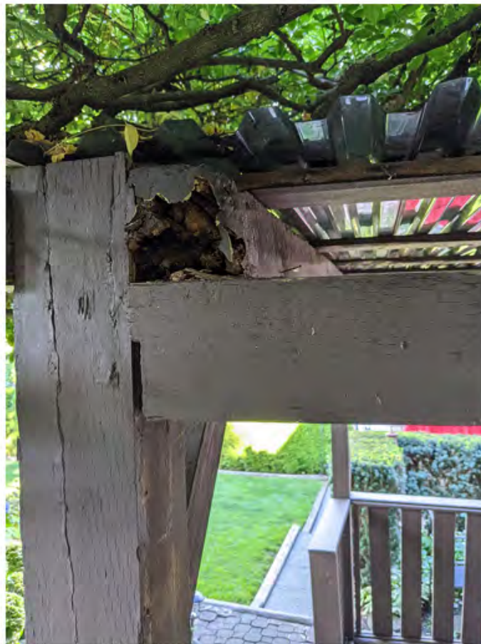
unit 349 - pergola with evidence of extensive rot.jpg
