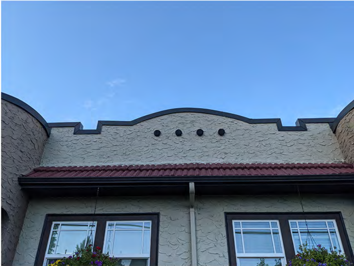
attic venting on south side.jpg
