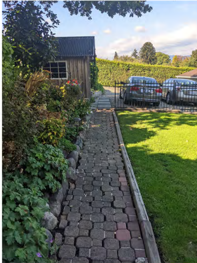
unit 349 - shifted paving stone path to shed and parking area.jpg
