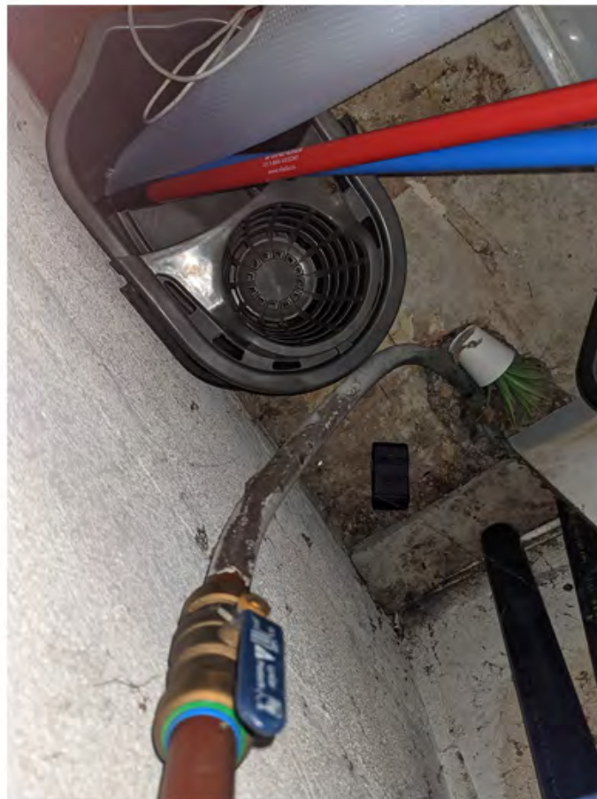
unit 349 - water supply to Subject Building with no meter and potential lead piping.jpg
