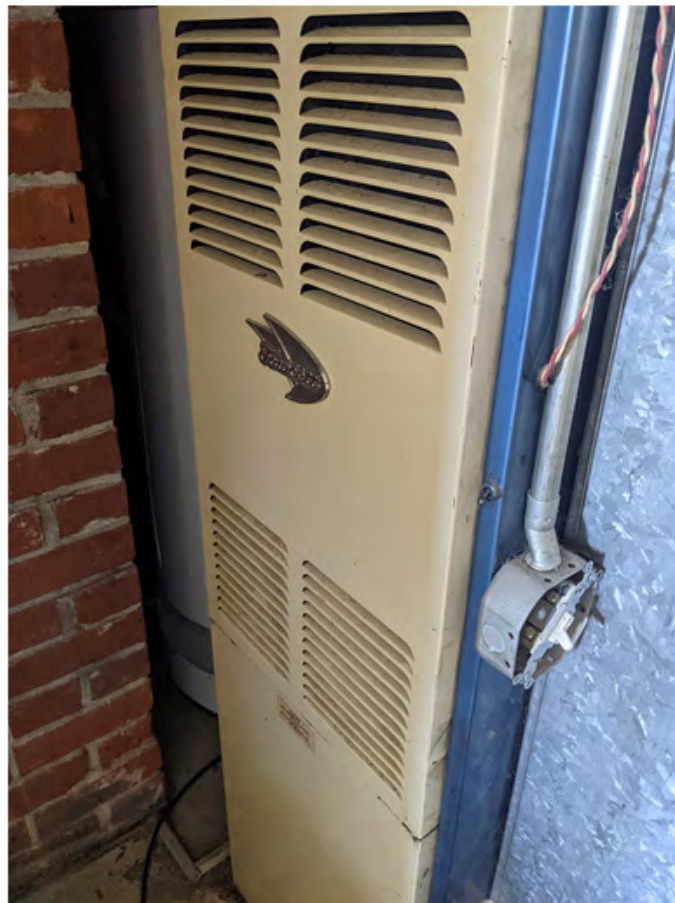
unit 349 - mid efficiency furnace likely at end-of-life with no replacement heat exchanger possible.jpg
