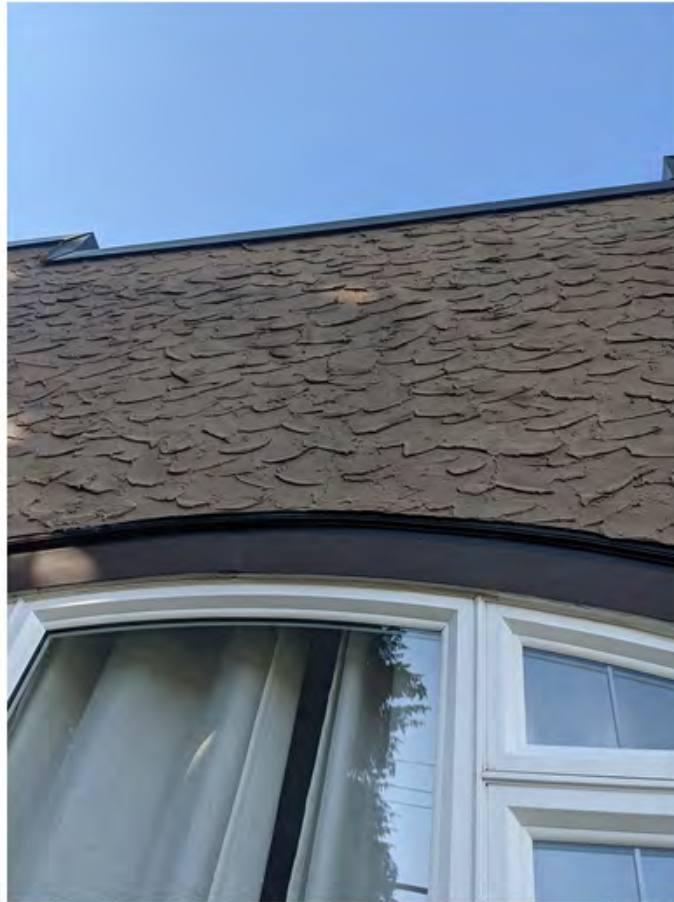
unit 349 - cracks in stucco above window.jpg
