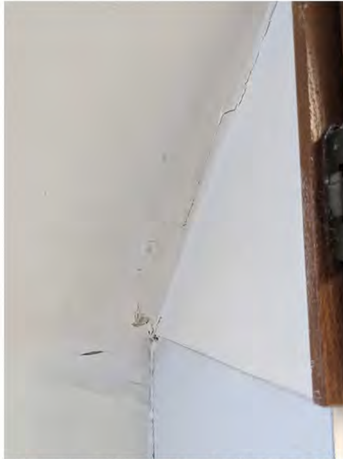
unit 349 - evidence of moisture ingress above stove in lower level likely from building envelope failure.jpg
