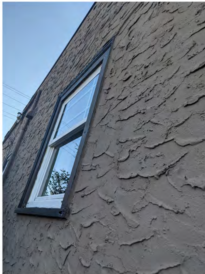
unit 349 - east wall window with no drip guard flashing above or below.jpg
