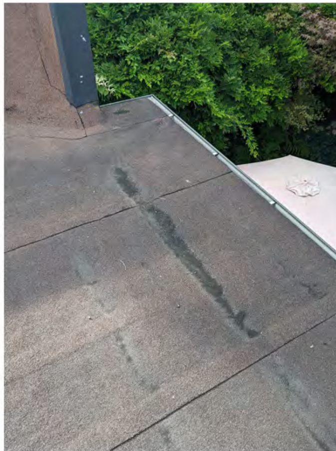
degraded rolled asphalt due to ice damming.jpg
