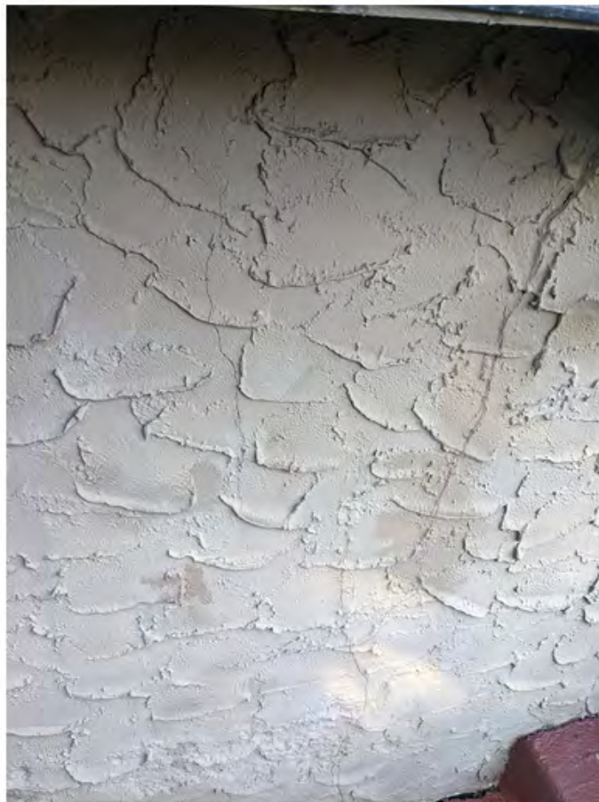
unit 349 - cracks in stucco on south wall justt west of entryway door.jpg
