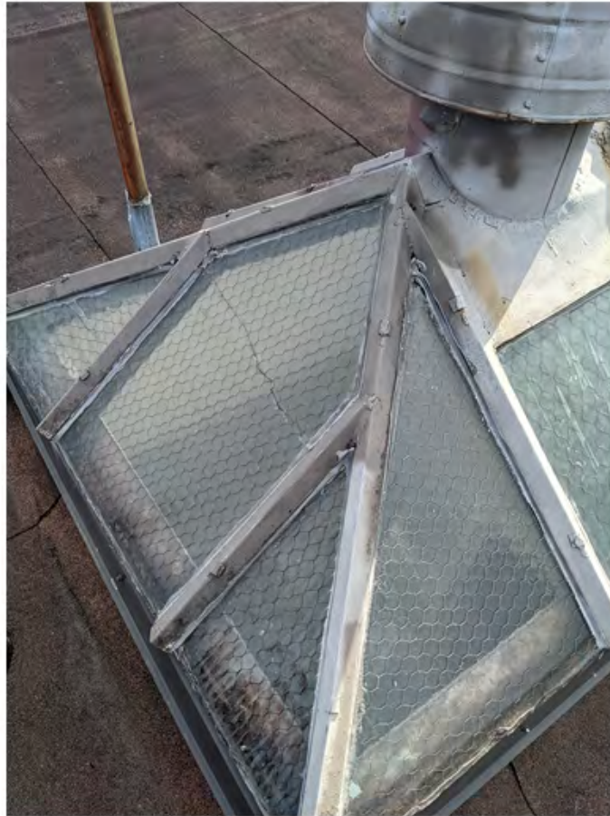
recent crack in skylight above unit 351.jpg
