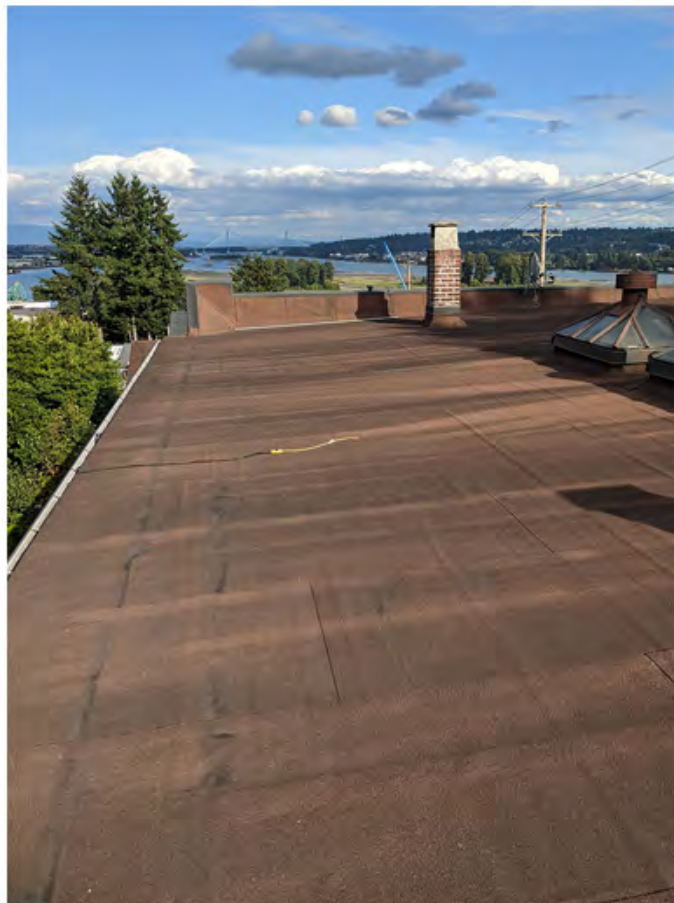
rolled asphalt no longer laying flat.jpg
