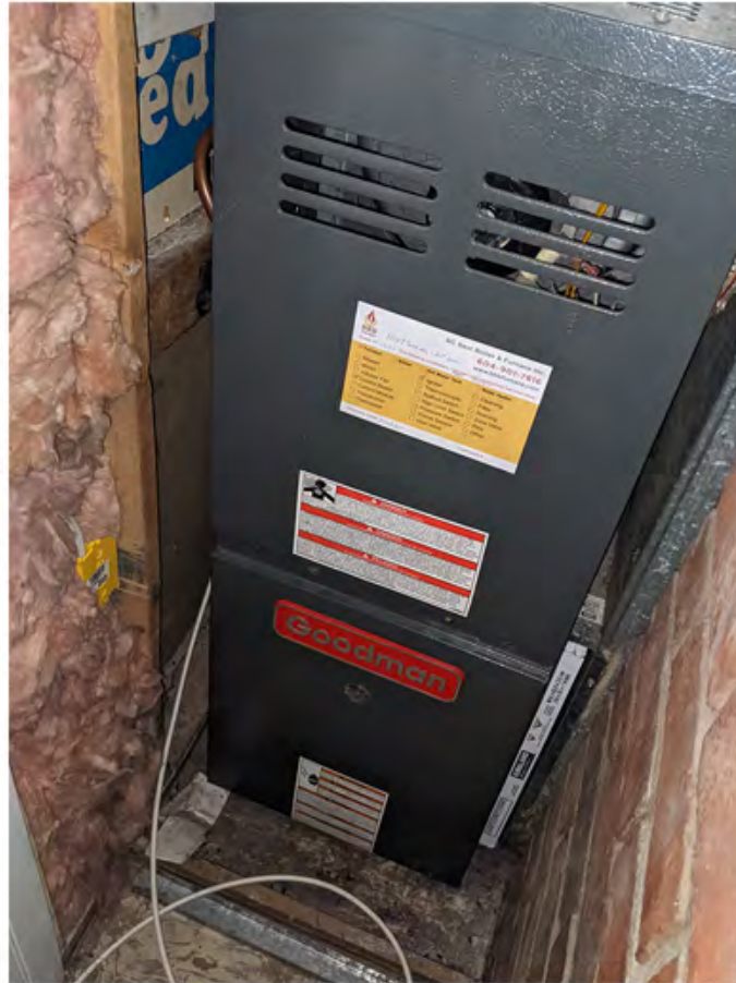
unit 351 - likely high efficiency goodman furnace.jpg
