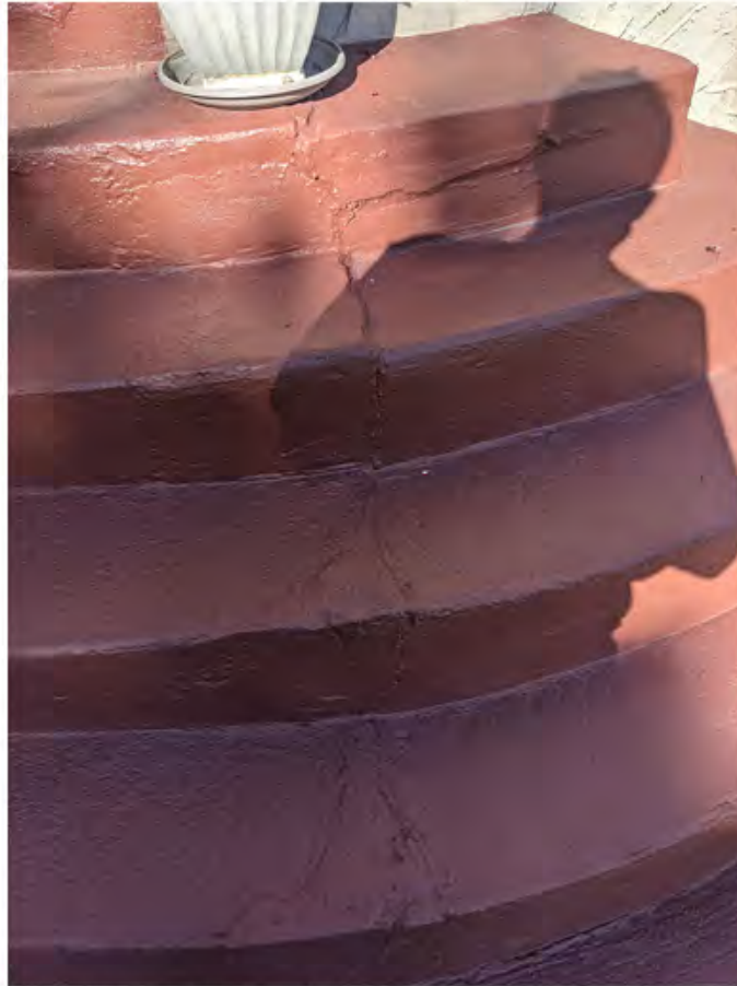
unit 349 - south entryway stairway cracks have increased in depth over the past 15 years.jpg
