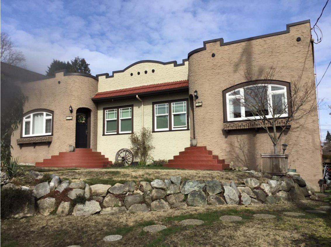
Figure 1: Current photograph of the front façade of 349 Cumberland Street
