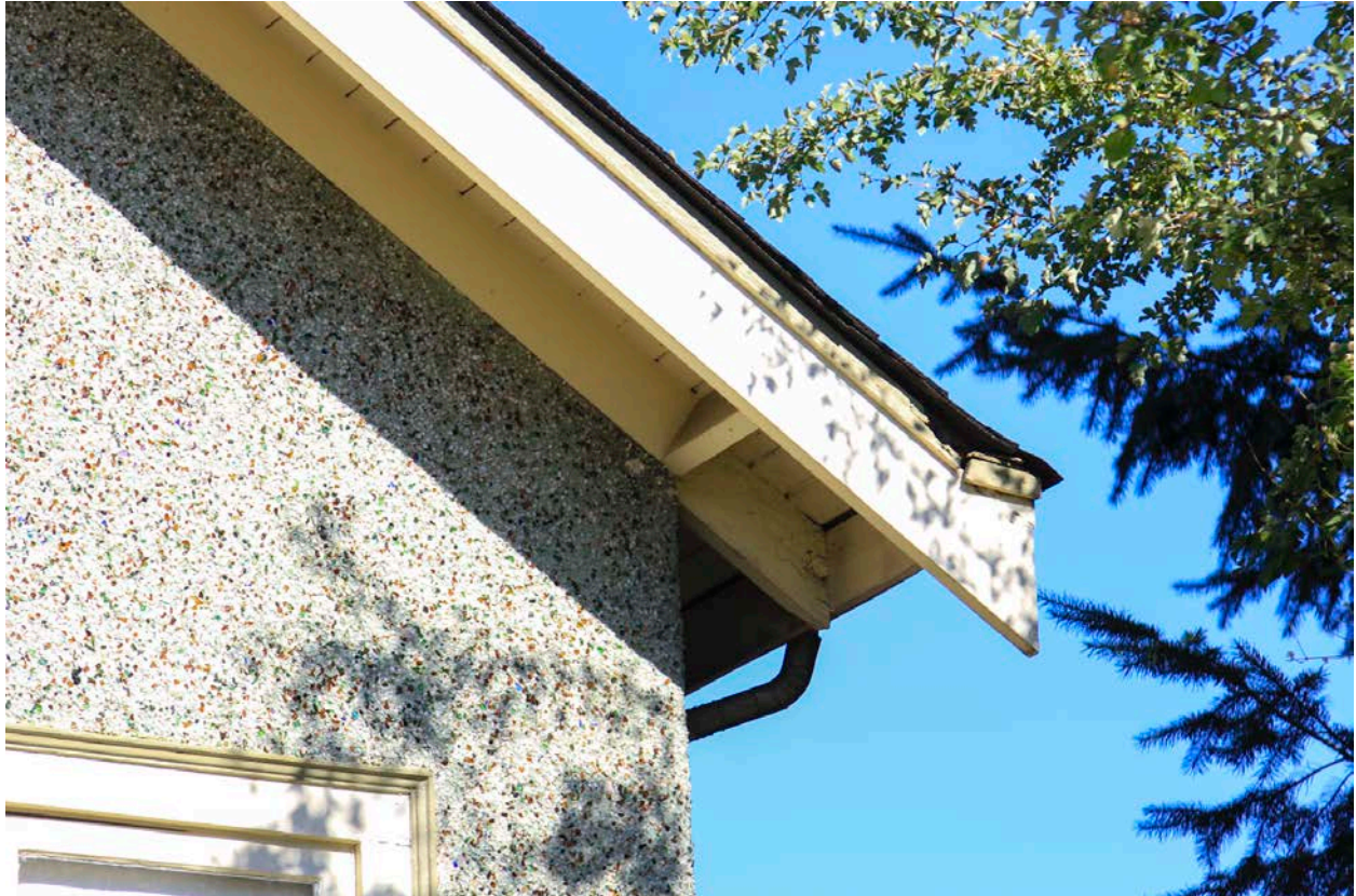
Detail of the front elevation gable showing the very small sprockets installed used to flare the bargeboard ends, Sept. 7, 2021. These sprockets are installed on the end of all bargeboards on the Morrow Residence.
