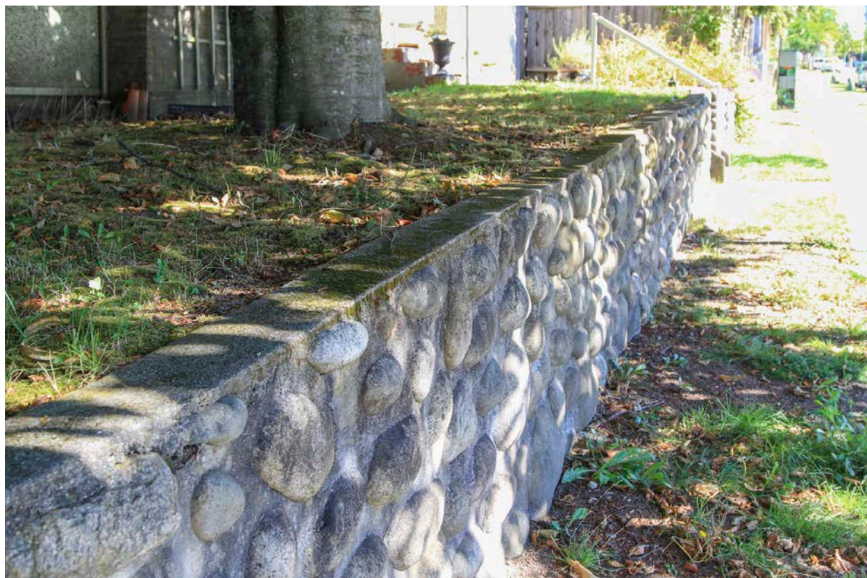
Detail of concrete and river rock retaining wall along Third Avenue, Sept. 7, 2021. Donald Luxton & Associates
