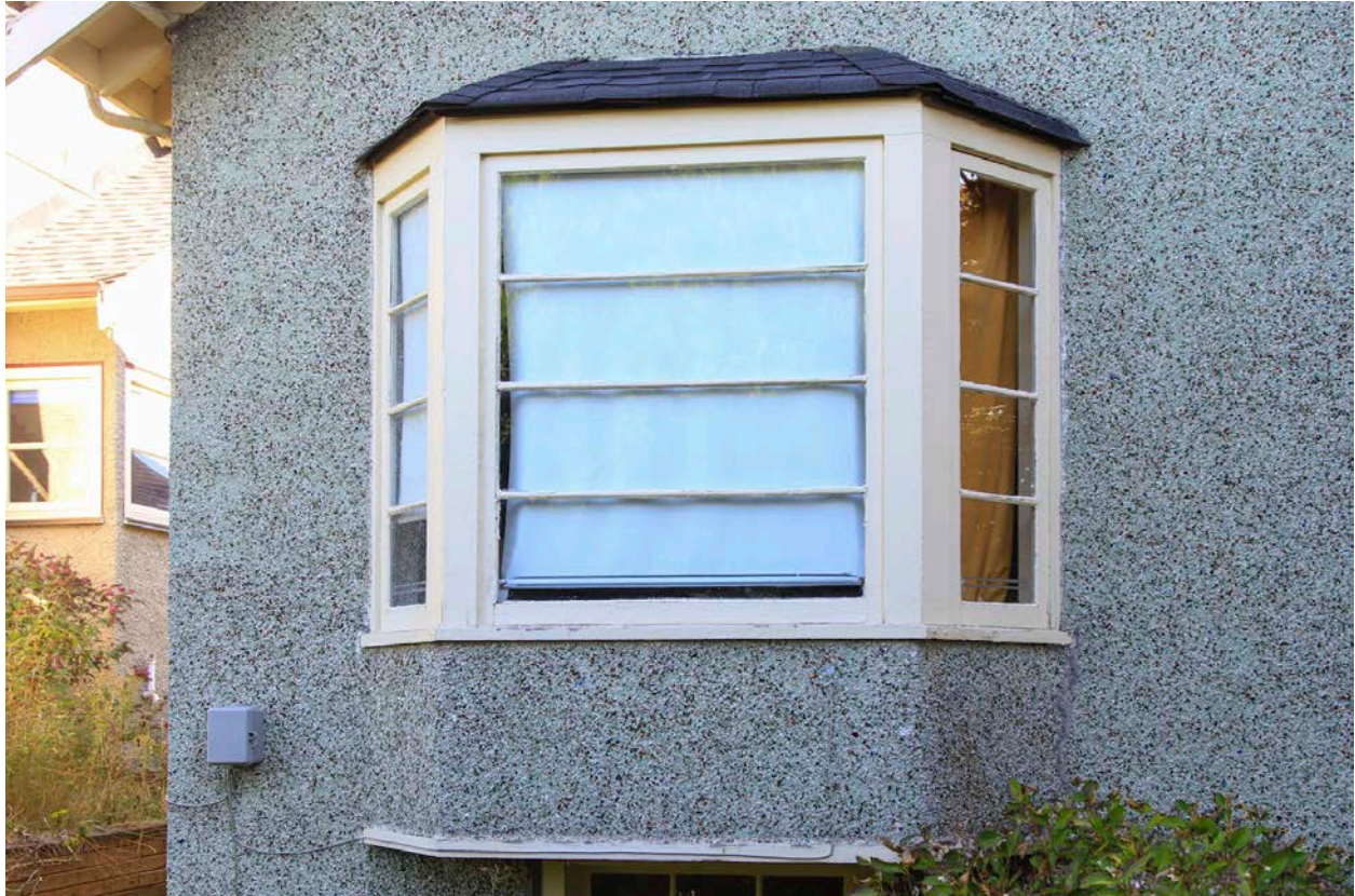
Detail of a canted oriel window on the southwest (Eighth Street) elevation of the Morrow Residence, Sept. 7, 2021.
