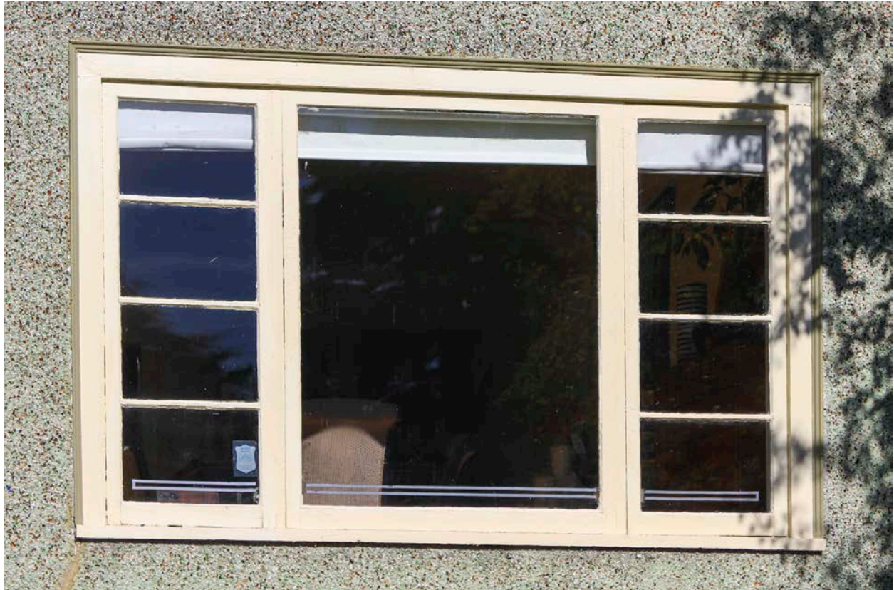
Detail of an original tripartite wood window assembly on the front elevation of the Morrow Residence, Sept. 7, 2021. All wood windows, with exception of the basement windows, feature horizontal muntins only.
