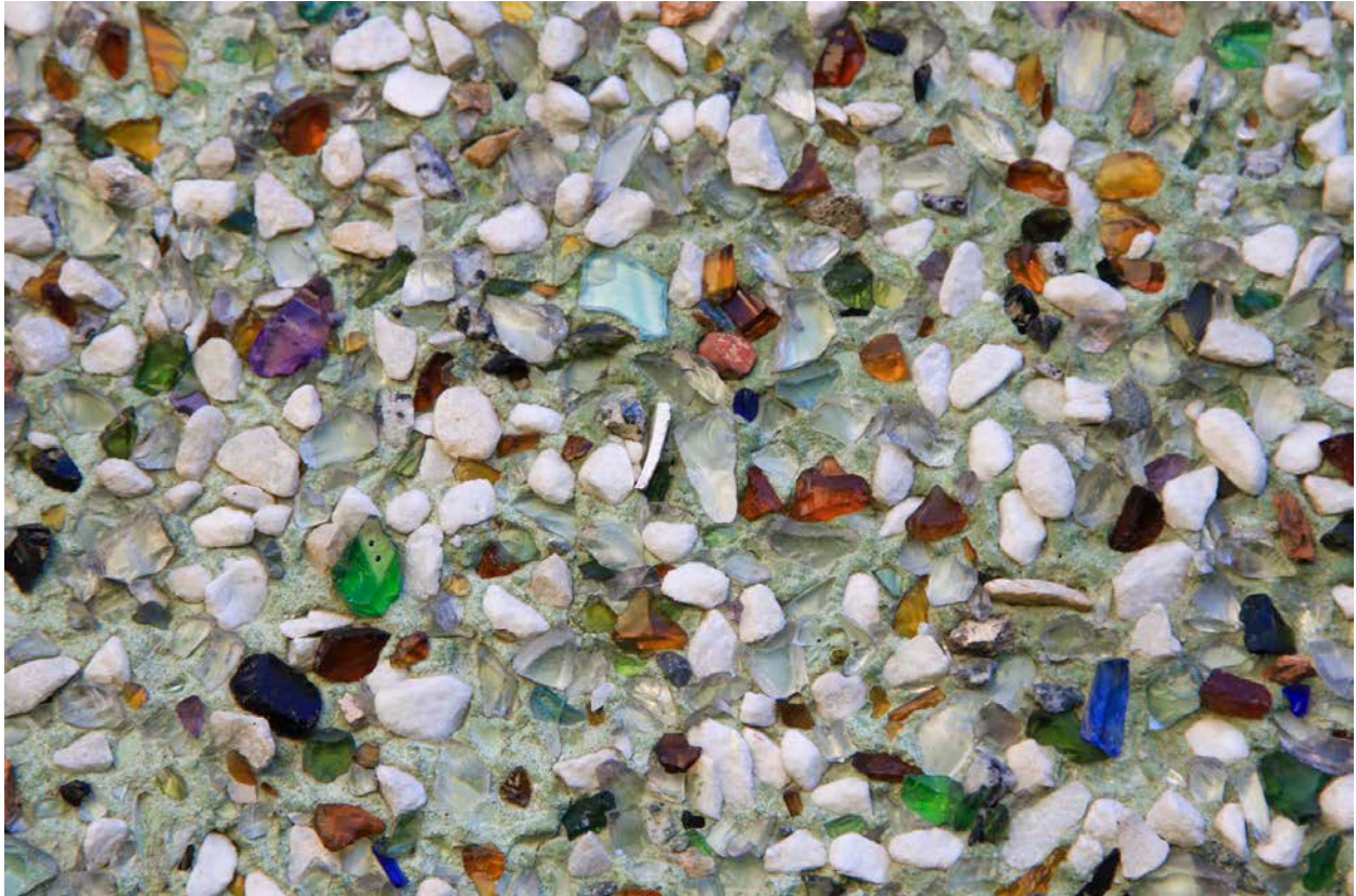
Detail of the original bottle dash stucco applied to the Morrow Residence, Sept. 7, 2021. Donald Luxton & Associates
