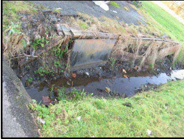
Existing non-standard wroughten wood lining ditch
