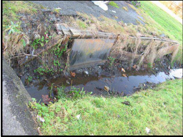
Existing non-standard wroughten wood lining ditch
