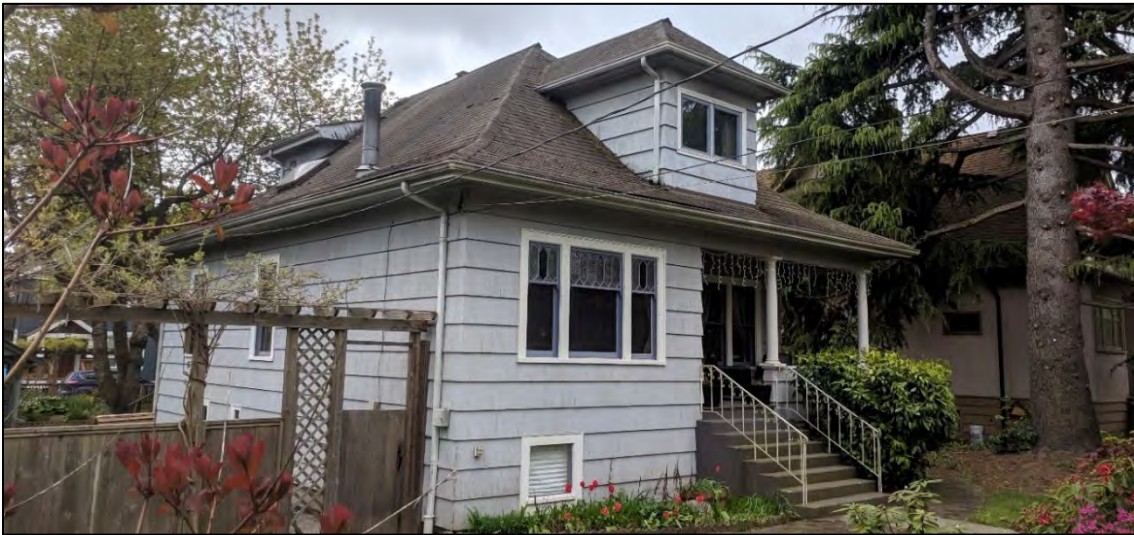
Fig. 15: Partial front and eastern side view of Calbicks House at 208 Fifth Avenue, 2019, illustrating its overall good condition. (Source: Cummer)
