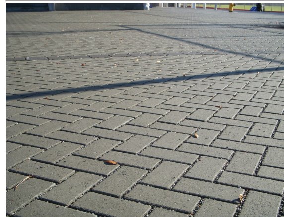
Permeable pavers for driveway
