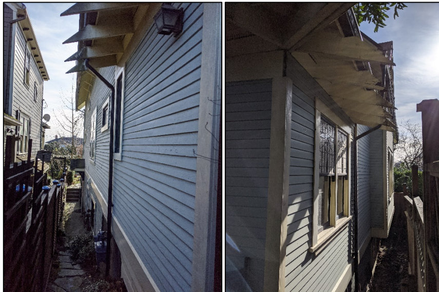
Figs. 9 and 10: Side views of Adams House at 515 St George Street. Left (Fig. 9) shows the eastern side and right (Fig. 10) shows the western side. (Sources: Cummer)
