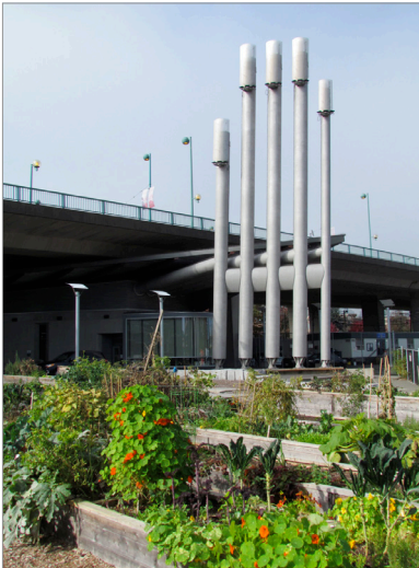
District energy system in City of Vancouver's Olympic Village neighbourhood.
