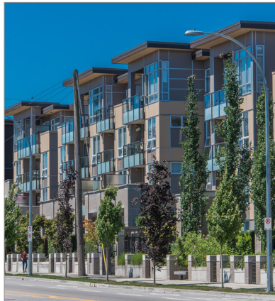
A low rise apartment building.
