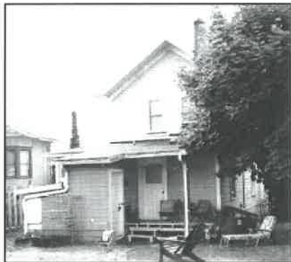
Photo of Rear Elevation 2009. Source: Basil Restoration
