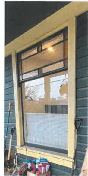
Front Elevation window, main level.
