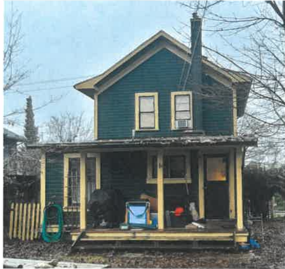
Project North - Rear Elevation
