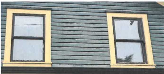
Front Elevation windows, upper level.
