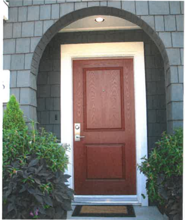
Example of simple, proportional details and material use at entry.
