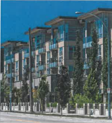
A low rise apartment building.
