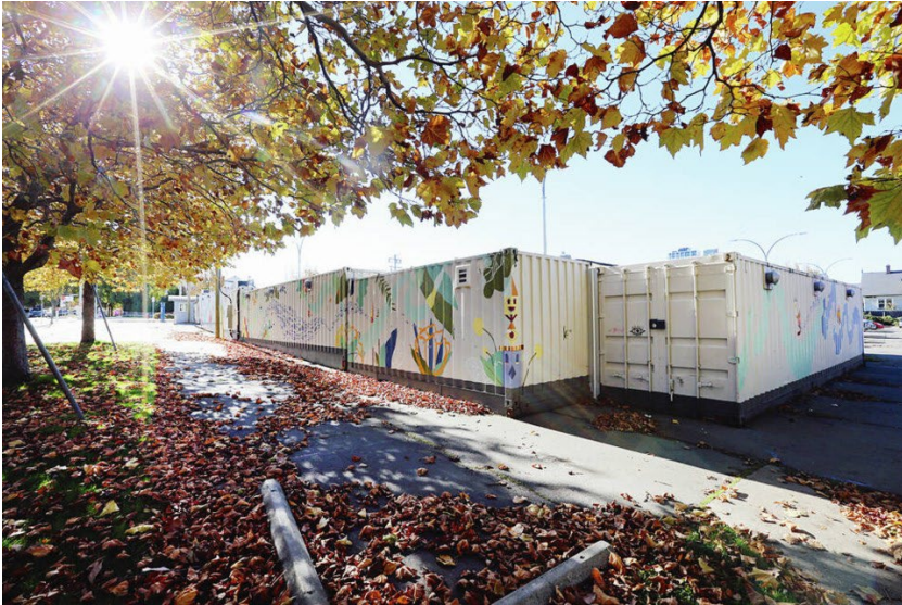
Exterior of containers, forming the walls of the village (Source: Adrian Lam, Times Colonist)
