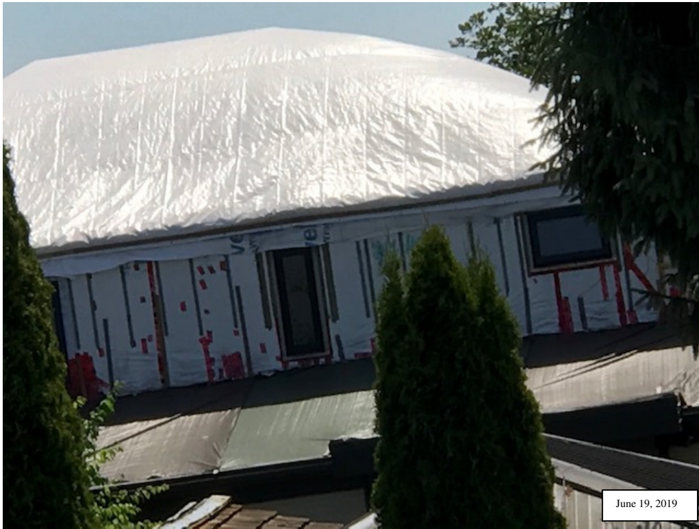
Pic 7: Rear elevation, showing roof tarped and unfinished cladding.
