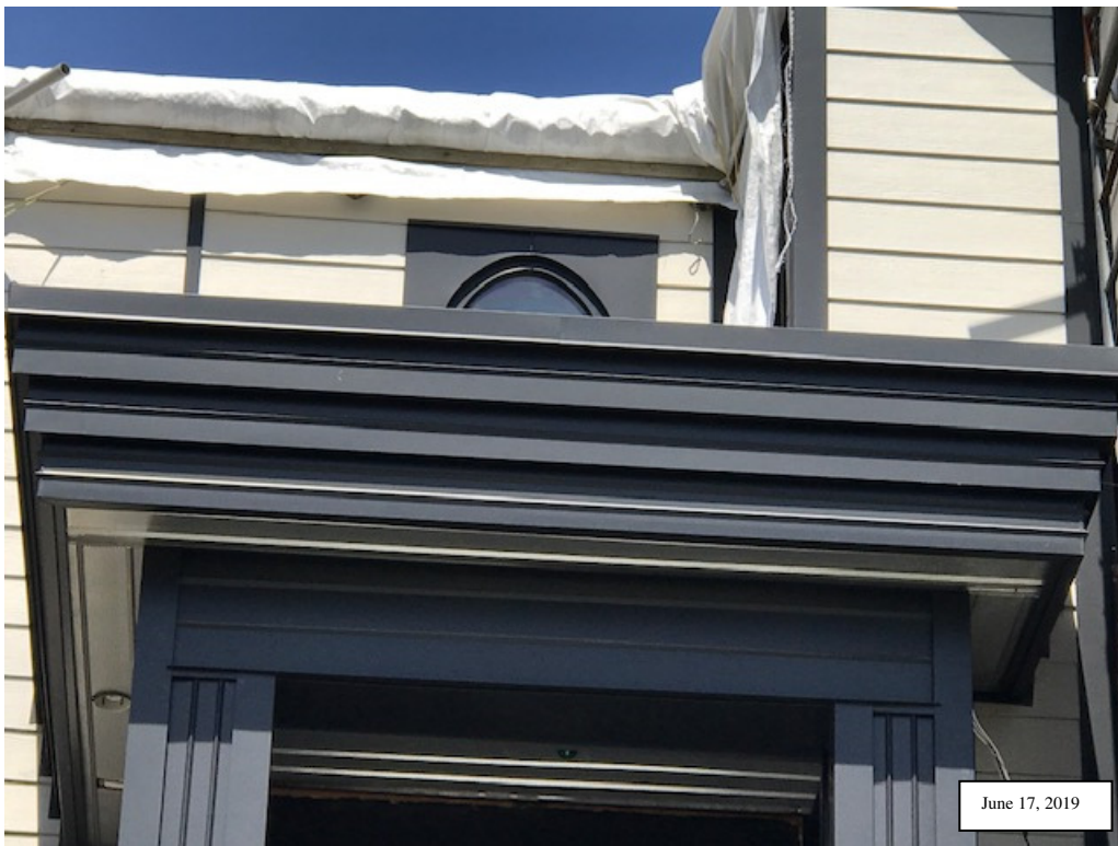
Pic 4: Front elevation showing upper deck without scupper to protect from flooding
