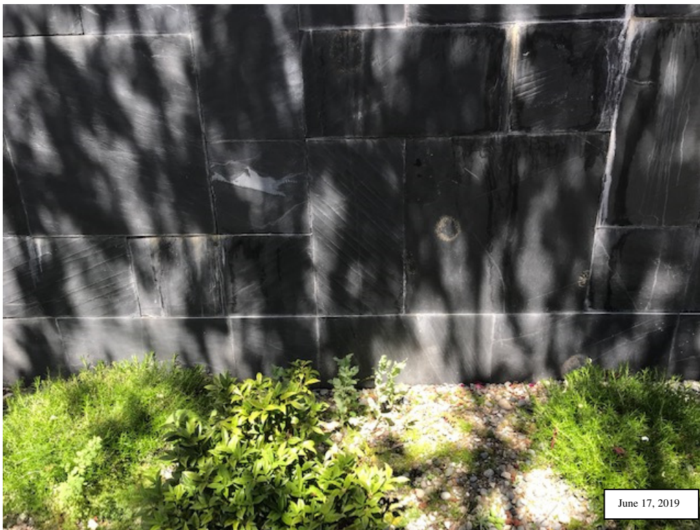
Pic 6: Front retaining wall showing tile has been installed over weeping holes. Note that there is no drain tile behind wall to relieve hydrostatic pressure. Overtime this may cause failure of the retaining wall.
