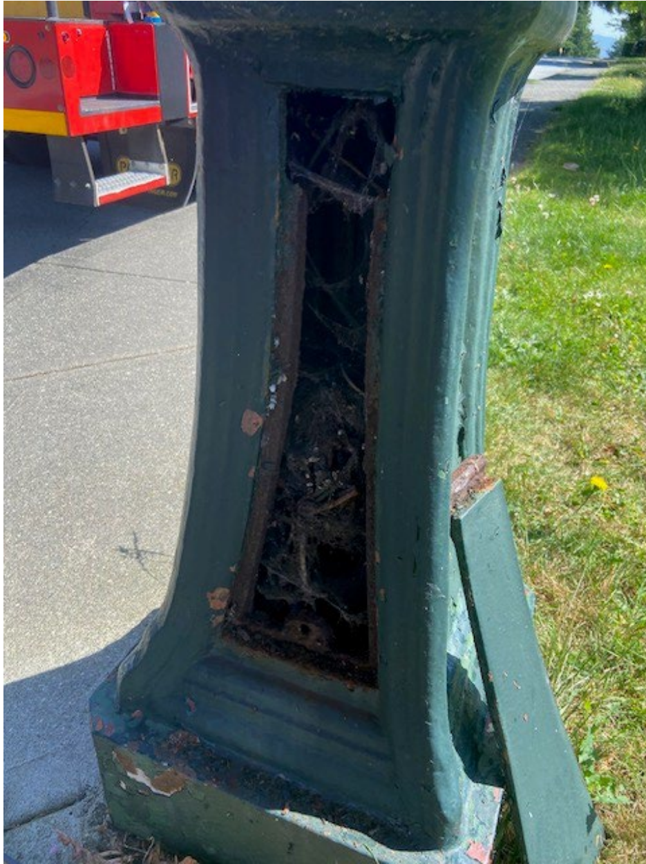
Typical base access hatch with inside metal corrosion
