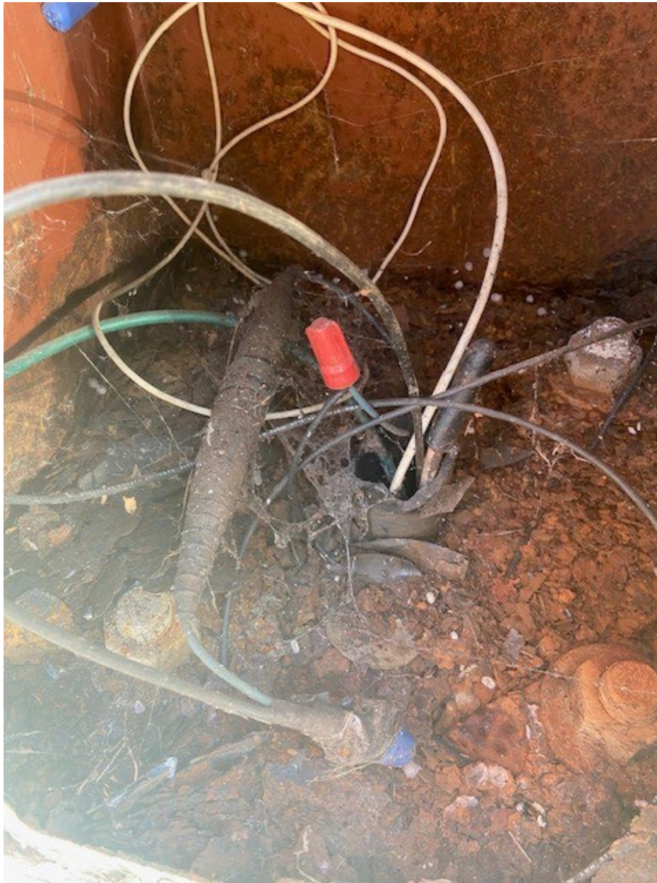
Inside hand hole view of the base top and heavy metal decay
