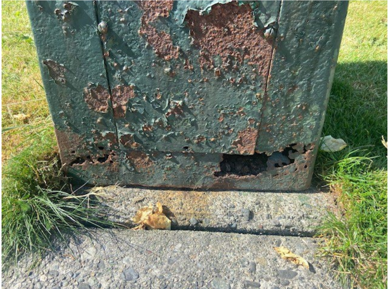
Different MVH style and the heavy metal decay
