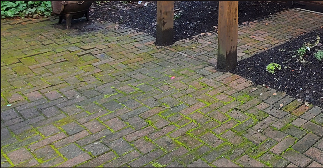
Fig. 29: View of some of the brick pavers at the back of Knott House at 318 Sixth Avenue, 2021, illustrating the various areas of moss growth. (Source: VanBrackel)
