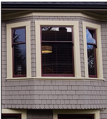
Figs. 26 and 27: Fig. 26 (left) shows the front horned wood window of Knott House, 2021. Right (Fig. 27) shows the western side with three other original horned wood windows as part of the second bay window closer to the back of the house. Note the good condition of these windows. (Source: VanBrackel)
