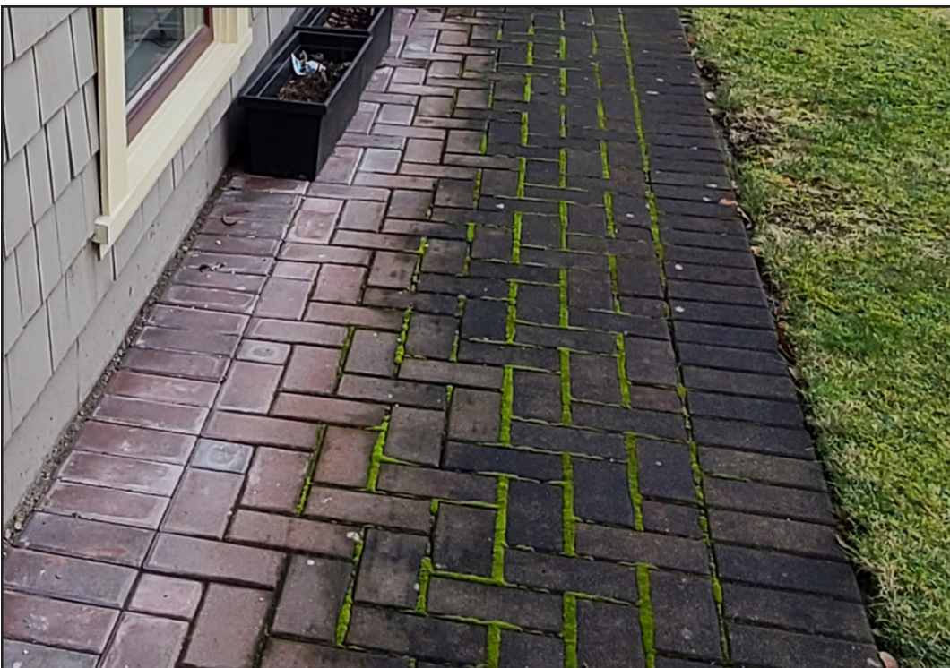
Fig. 30: View of some of the brick pavers along the western side of Knott House at 318 Sixth Avenue, 2021, illustrating additional areas of moss growth. (Source: VanBrackel)
