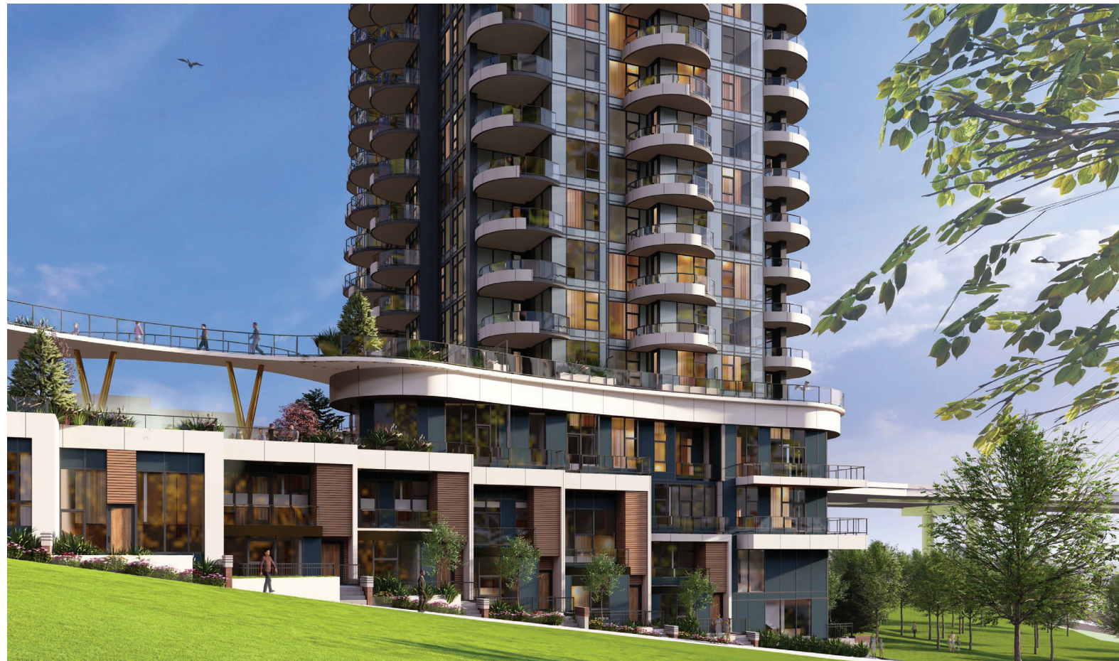
Podium view along Albert Crescent Park
