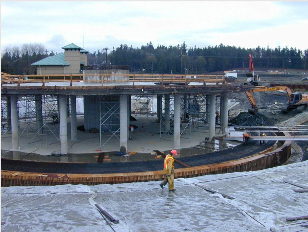
Cloverdale Sanitary Sewer Overflow Storage Tank under construction in Surrey
