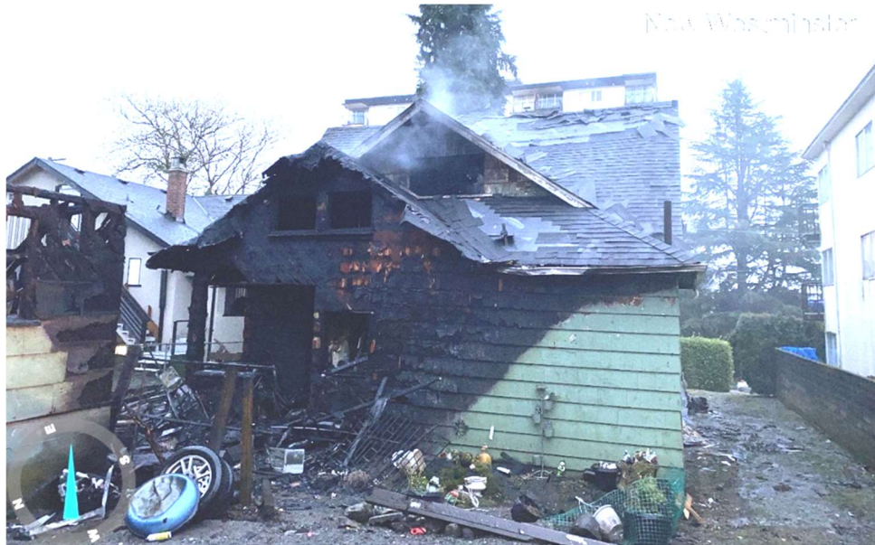
Figure 1: Rear of the house located at 707 Queens Avenue.
