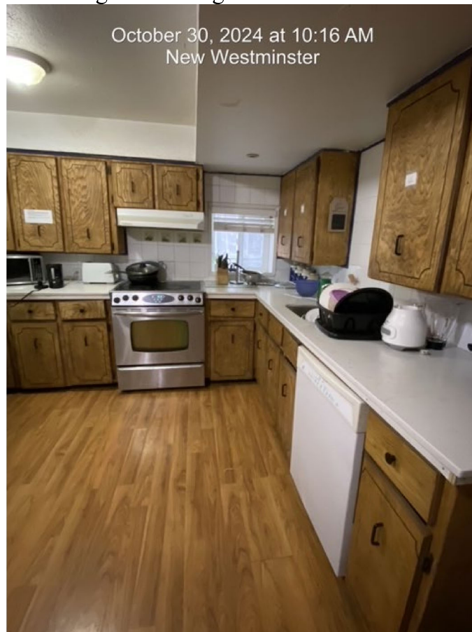
Photo 5 – Image of lower ground level kitchen at dwelling
