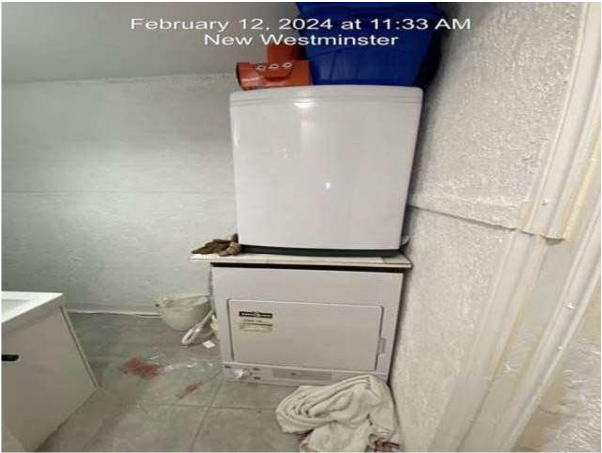
Pic 31 – second floor north entry bathroom bachelor unit
