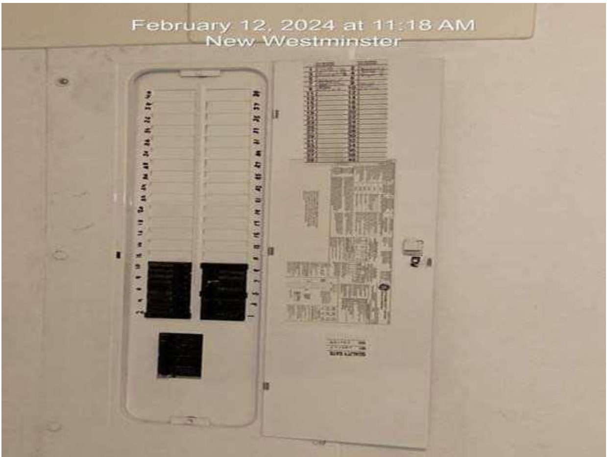
Pic 14 – ground level unit – space heaters used for heat
