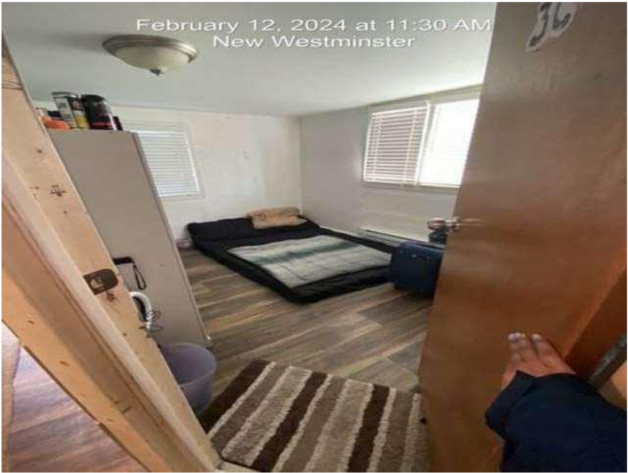
Pic 26 – ground level rear entry unit bedroom
