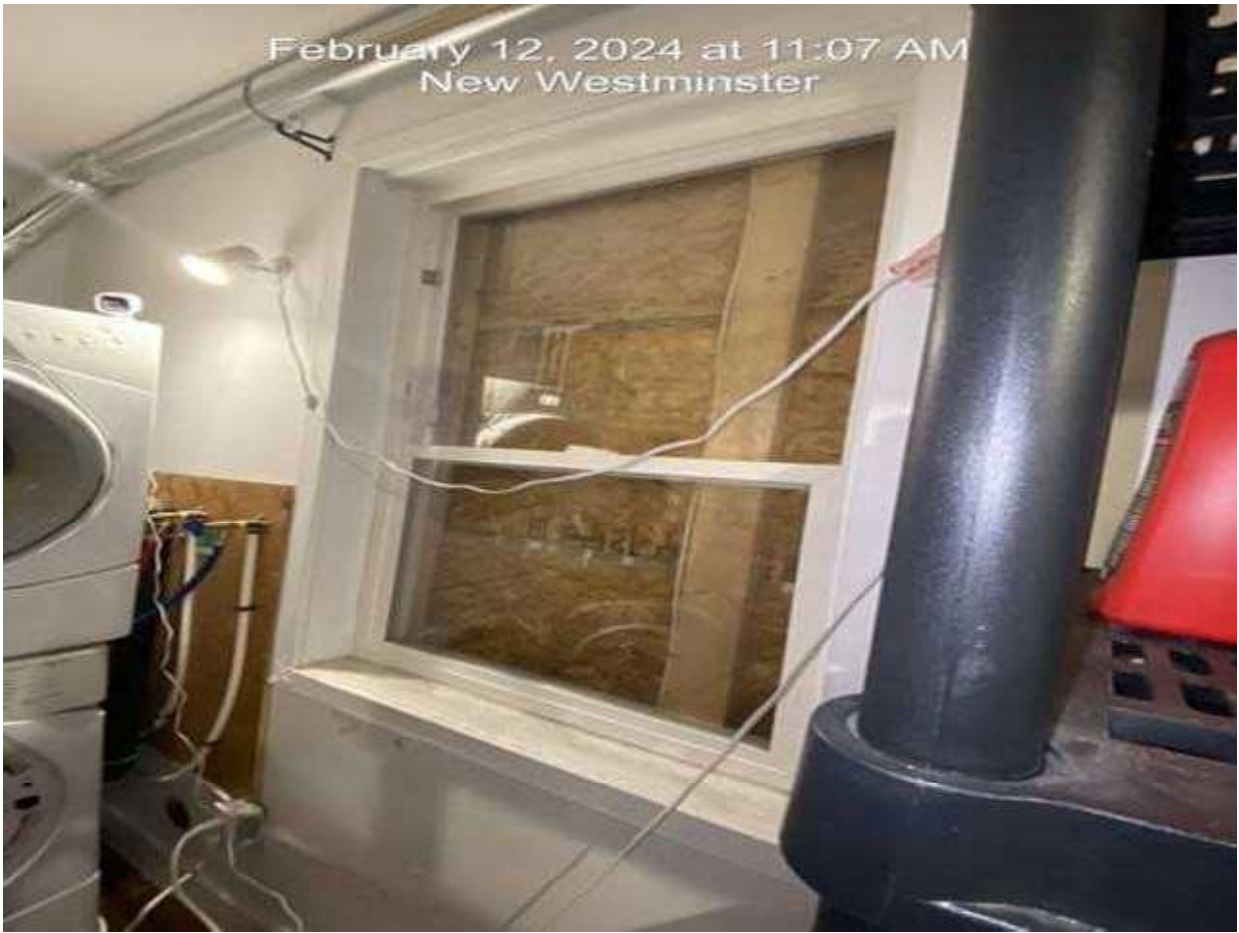
Pic 6 – second floor bathroom
