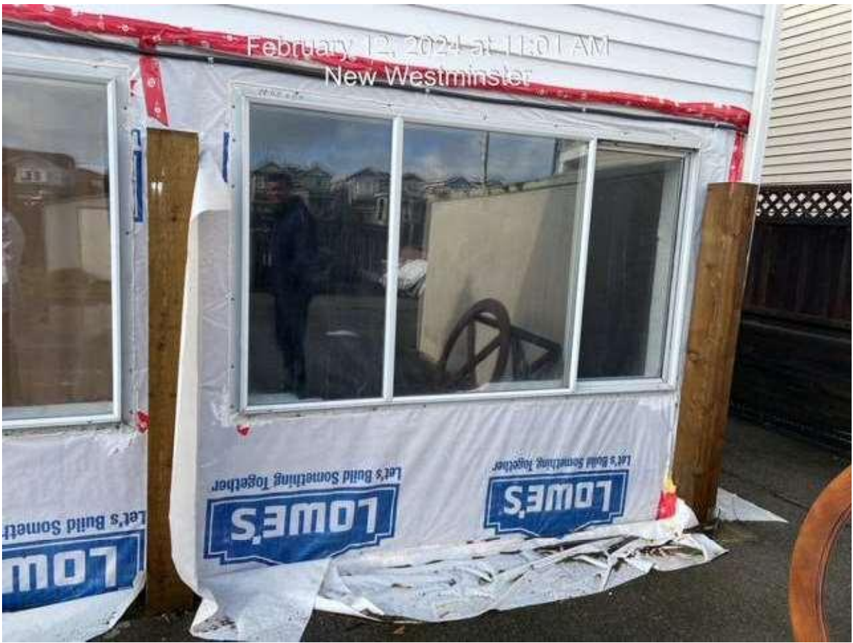
Pic 2 – work conducted at rear of the property
