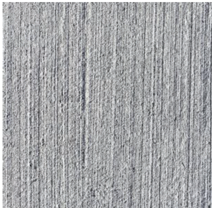
CONCRETE PAVING BROOM FINISH
