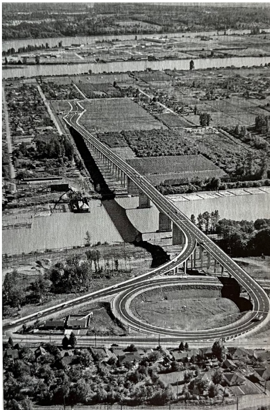
Figure 11: Newly completed Queensborough bridge, c. 1960. Source: Royal City , Jim Wolf, Heritage House Publishing, 2005.
