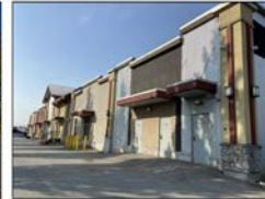
EXISTING RETAIL BUILDING – NORTHEAST ELEVATION
