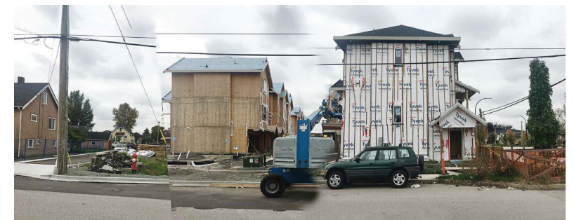
VIEW WEST OF TOWNHOUSES AT EWEN AVE. & PEMBINA ST.
