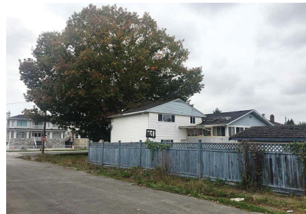
VIEW OF SITE WEST FROM SALTER ST.
