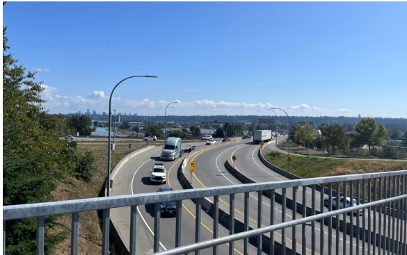
Multiple Jurisdictions In addition to being on unceded Coast Salish territory, multiple jurisdictions have a presence in the neighbourhood, including the Ministry of Transportation and Infrastructure, TransLink, and BC Hydro. The area is also bordered by the City of Burnaby.
