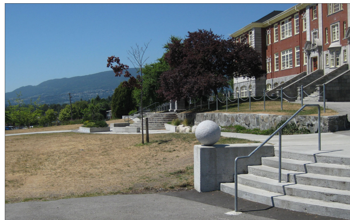
CONCRETE STAIR - SEATWALLS DESCRIPTION: CAST IN PLACE CONCRETE, WITH SEATWALLS SANDBLAST FINISH, HAND RAILS
