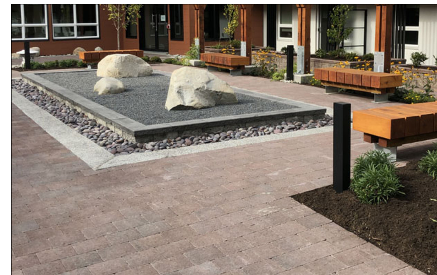
CONCRETE UNIT PAVERS FOR WALKWAYS DESCRIPTION: CONCRETE UNIT PAVERS SOLDIER OR RUNNING BOND PATTERN
