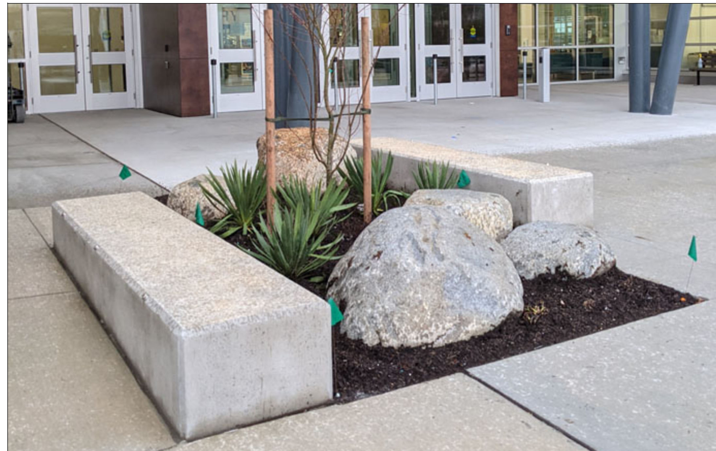
CONCRETE SEATWALL DESCRIPTION: CAST IN PLACE CONCRETE, SANDBLAST FINISH WITH SKATEBOARD DETERANT
