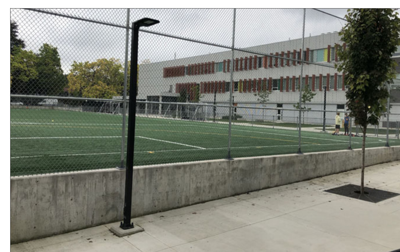
CHAIN LINK FENCE FOR SPORTS FIELD DESCRIPTION: ALL WELDED GALVANIZED STEEL CHAIN LINK FENCE
