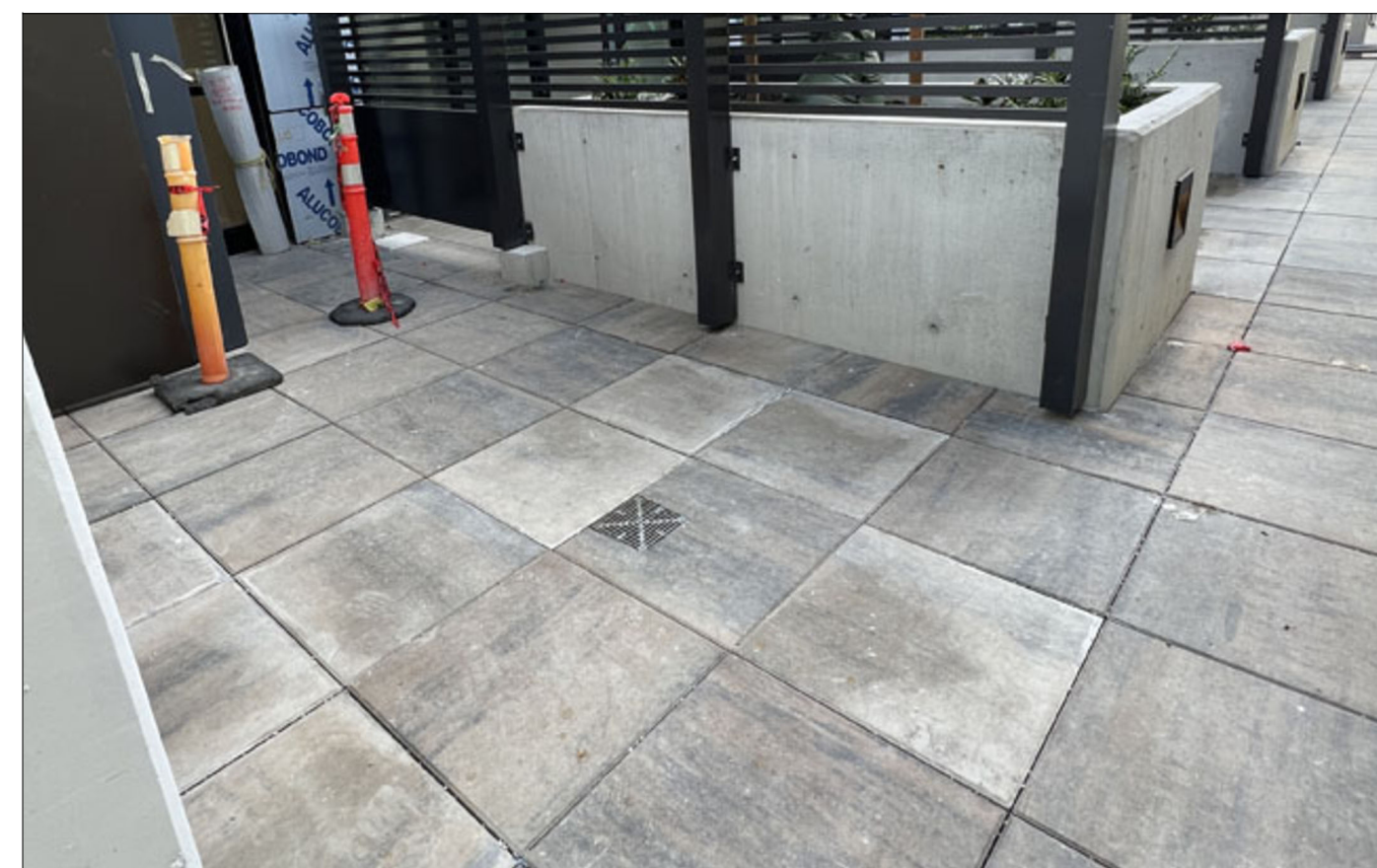
CONCRETE UNIT PAVERS FOR PATIOS DESCRIPTION: 600X600 (2'X2') CONCRETE UNIT PAVERS WITH PLASTIC PEDESTAL
