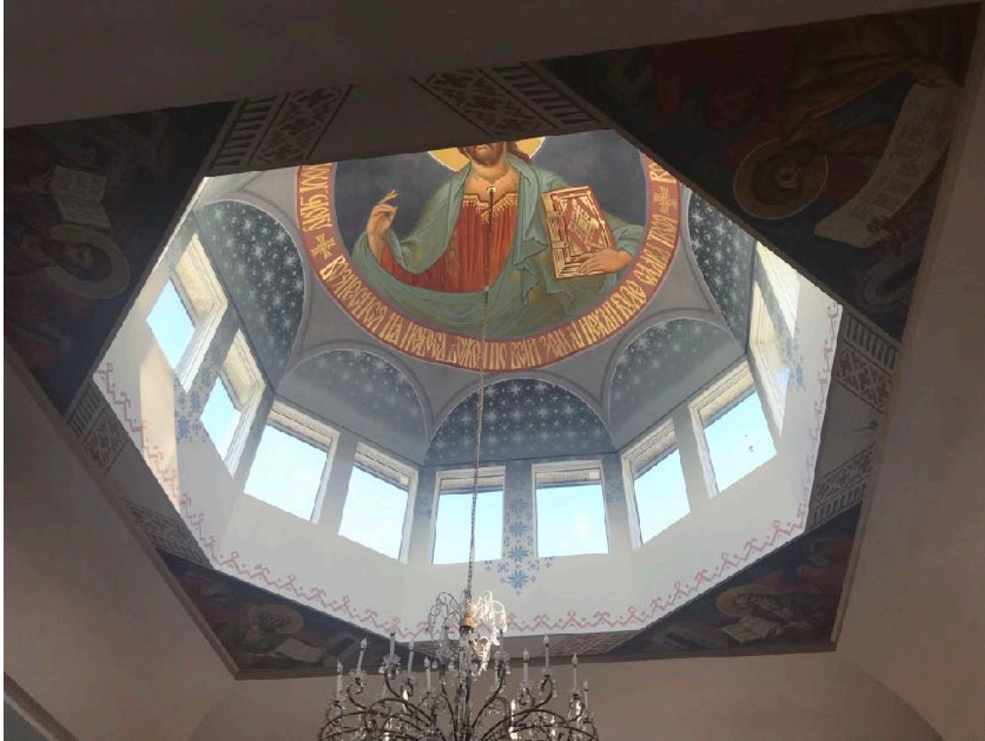
View of dome interior and clerestory windows
