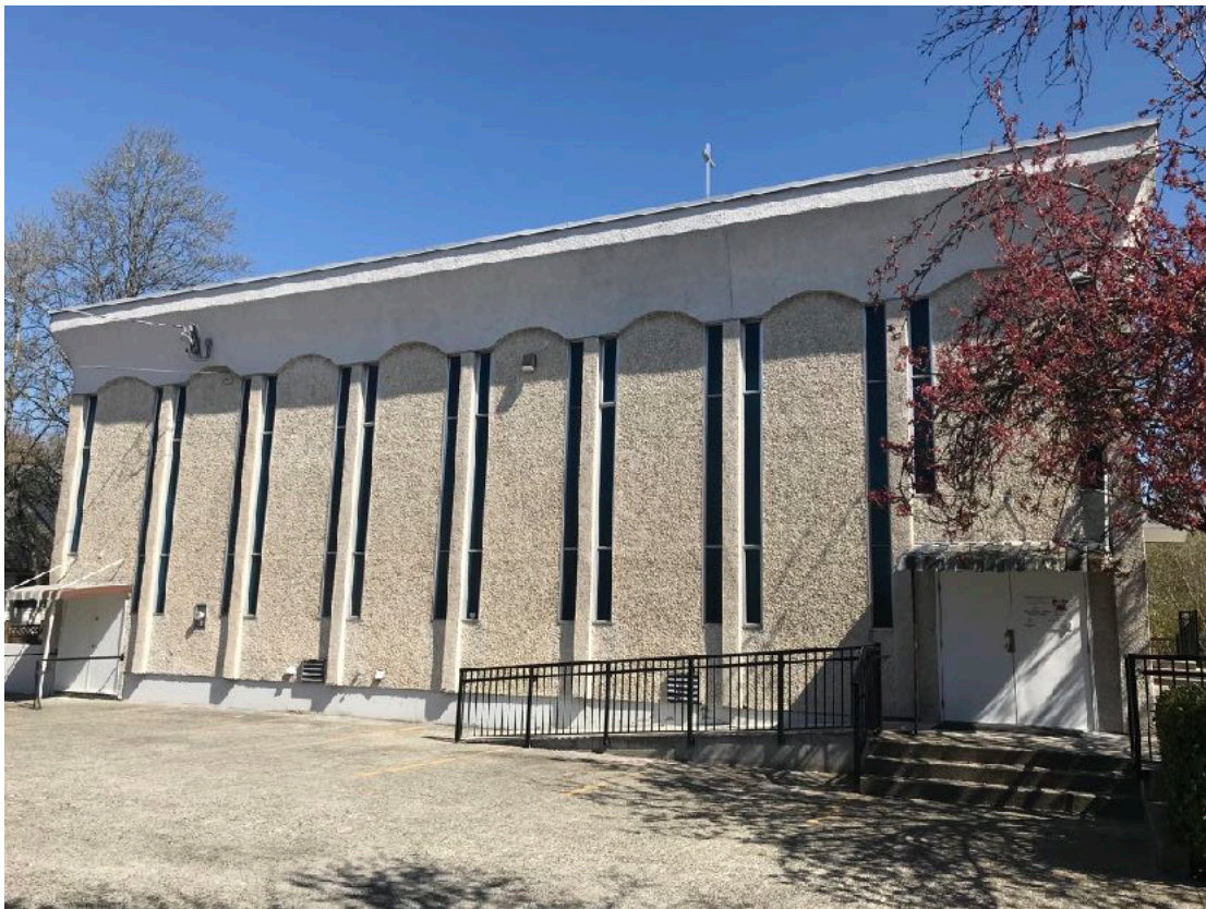
Side view (facing parking lot)
