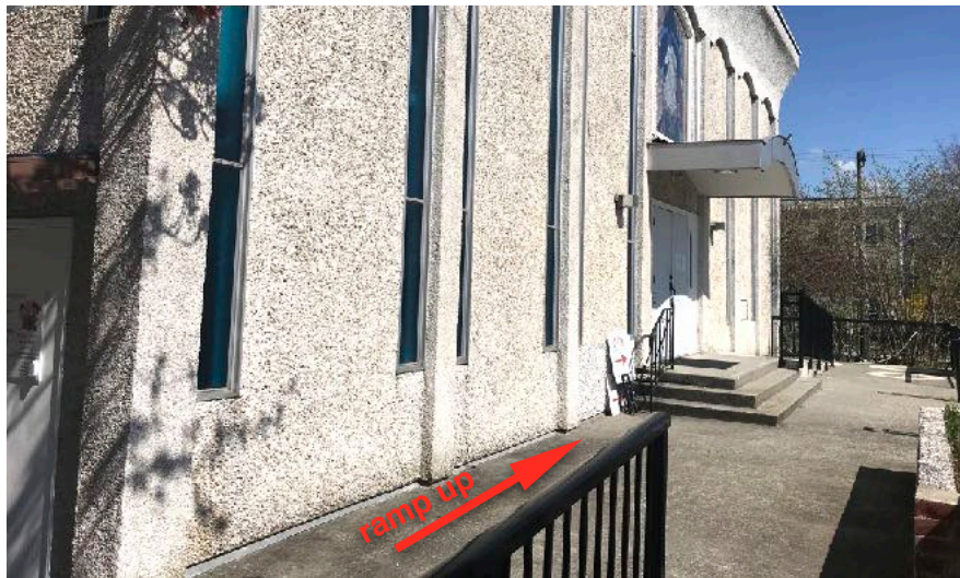
Photo showing the last section of the 'accessibility ramp' arriving at the entrance podium but more stairs at the church entrance doors are left to tackle.
