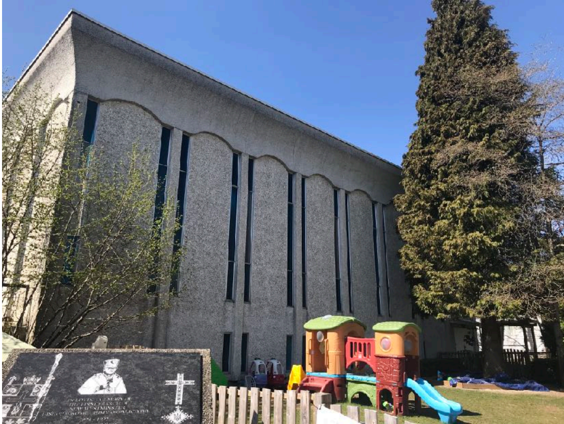
Side view (facing 5th Street)
