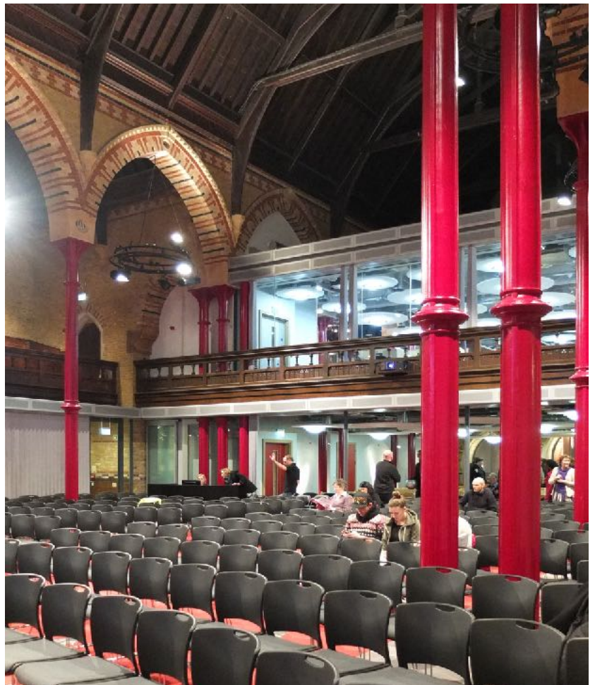
Photograph of the rehabilitated choir loft in St. Jude's Church in Kensington, London. The loft is not only closable with sliding glass doors but an extra layer of blinds can be pulled down to give visual separation. Source: Ellis and Moore Consulting Engineers
