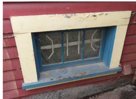
The only original window - at grade on the north elevation.
