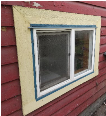
Example of new window insert and wood casing.
