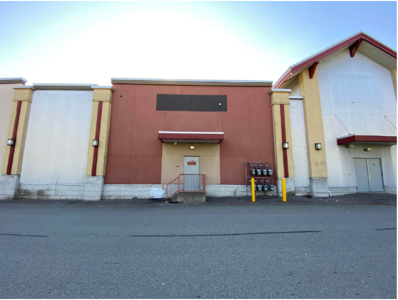
8 VIEW LOOKING WEST A105 NTS
