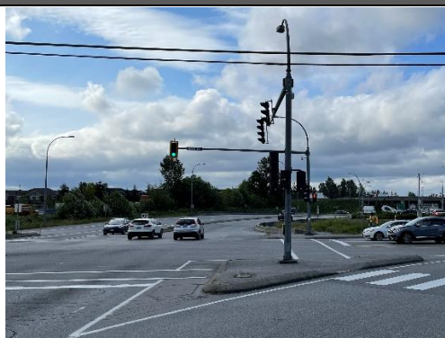
Southbound Approach – facing south (only one signal head for two through lanes)
