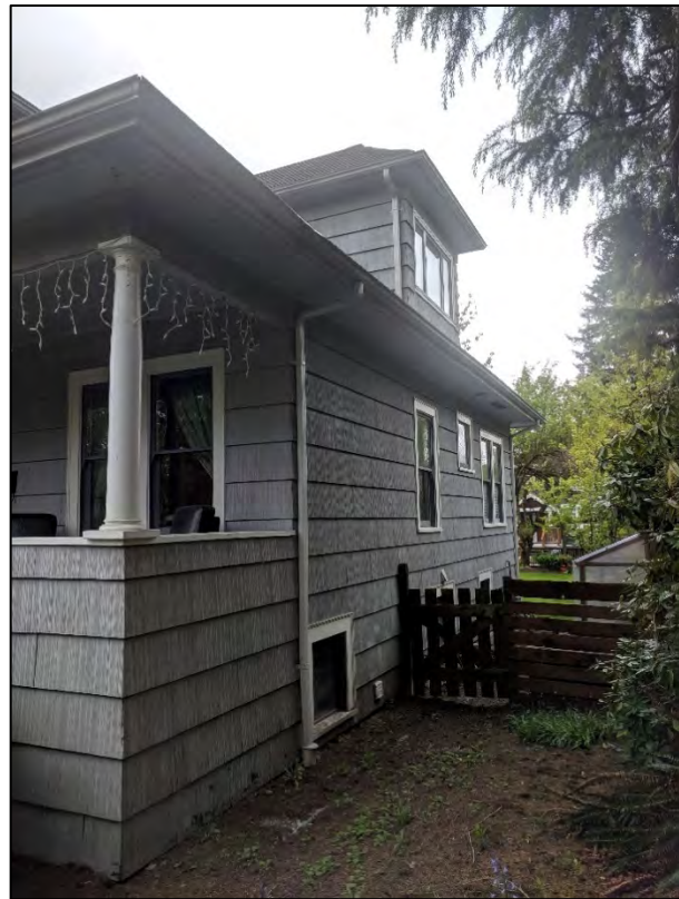
Figs. 11 and 12: Western side view of Calbicks House at 208 Fifth Avenue, 2019, from the back (left, Fig. 11) and the front (right, Fig. 12). Note the double-hung horned wood windows and the square wood windows. (Sources: Cummer)
