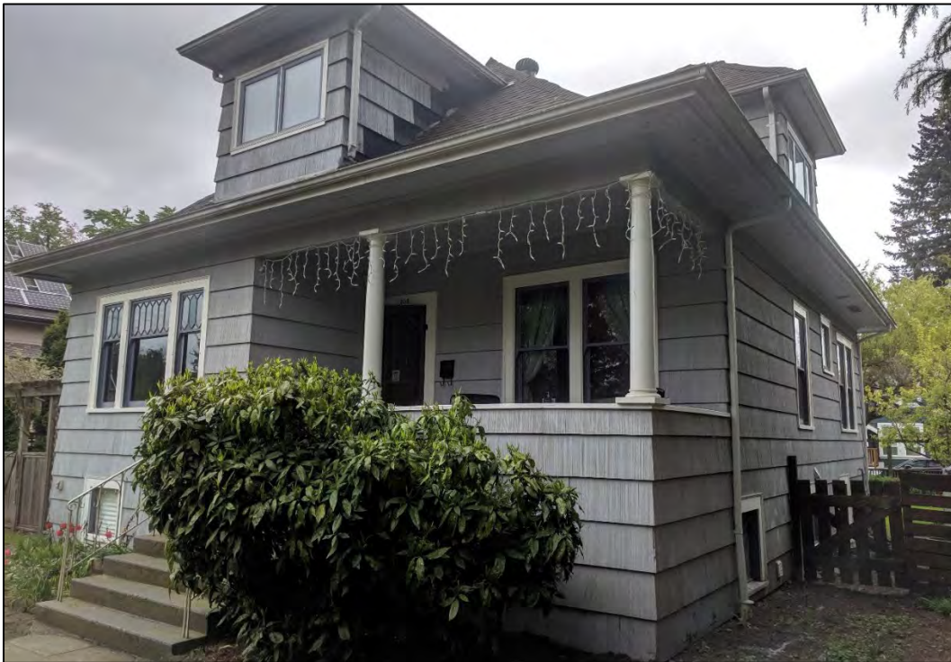
Fig. 19: Northwestern front and side view of Calbicks House at 208 Fifth Avenue, 2019, illustrating the overall good condition of its exterior wood elements. Note the landscaping possibly growing too close to the foundations, as discussed in section 9.9 below. (Source: Cummer)
