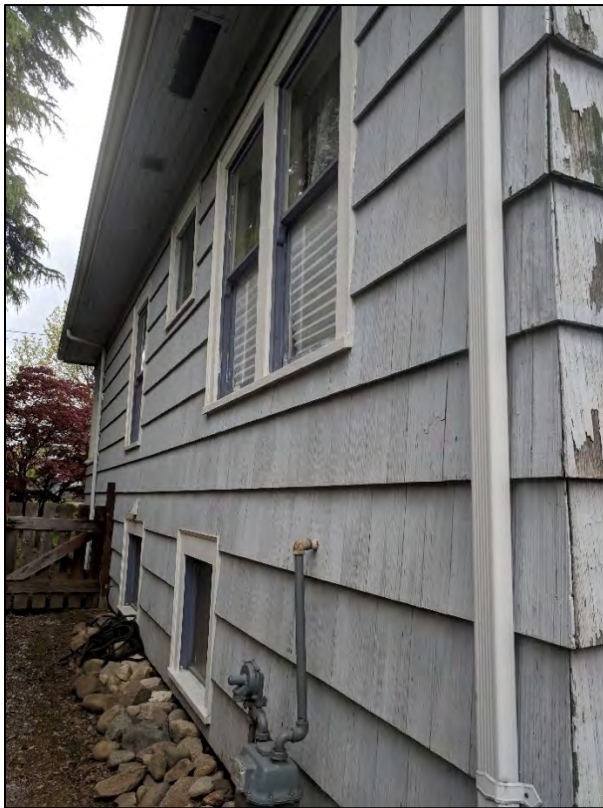
Figs. 11 and 12: Western side view of Calbicks House at 208 Fifth Avenue, 2019, from the back (left, Fig. 11) and the front (right, Fig. 12). Note the double-hung horned wood windows and the square wood windows. (Sources: Cummer)
