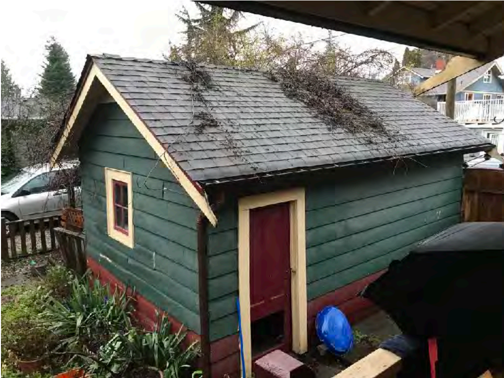
Garage structure viewed from inside the house
