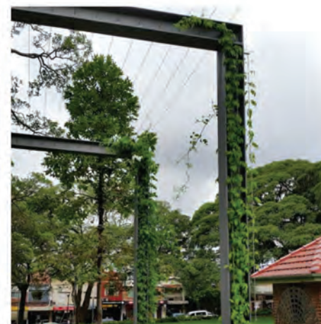
OVERHEAD CABLE TRELLIS
