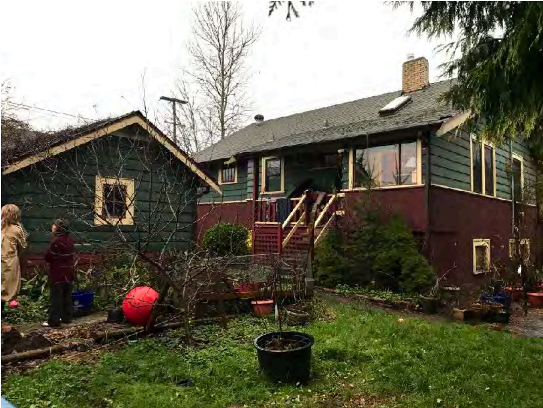
Side and rear view showing rear of garage
