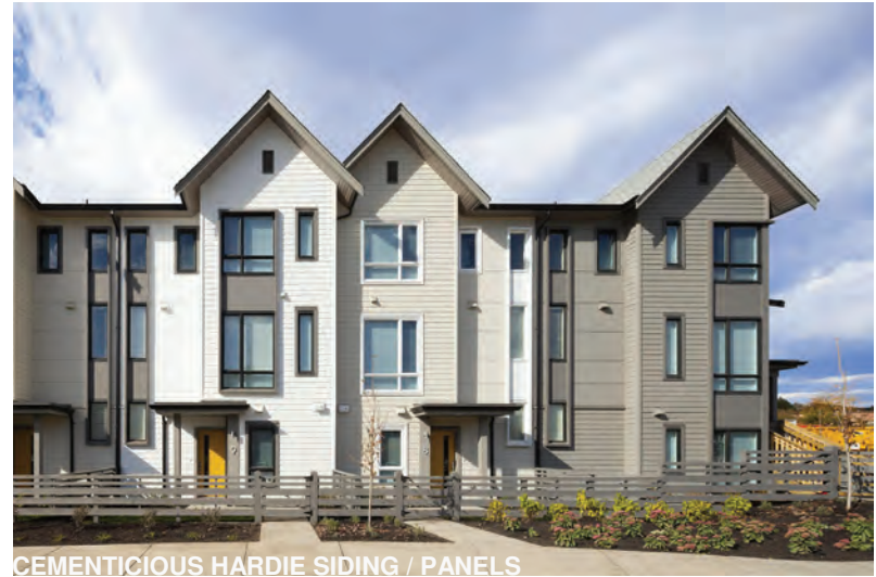
CEMENTICIOUS HARDIE SIDING / PANELS
